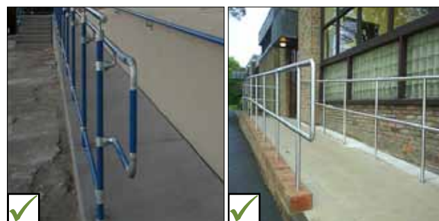
Figure 7b: Handrail Returns to Wall
