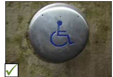
Example of circular power door operator control.
