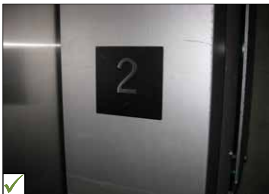
Tactile elevator car identification sign.
