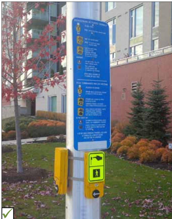
Typical APS actuation.
