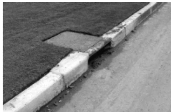
Curb-face type inlet are not obstacles to road users, especially cyclists.
