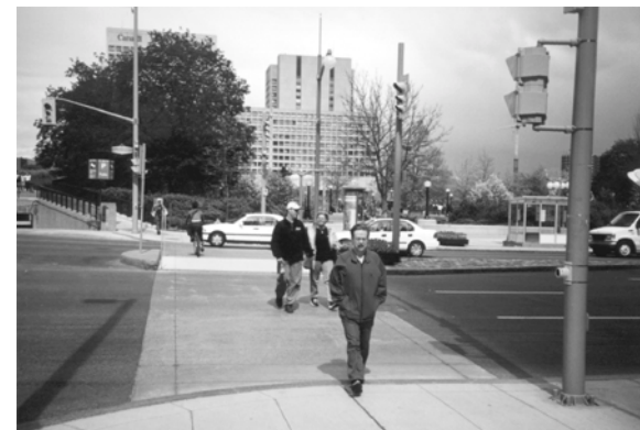
Special paving can be used to delineate the pedestrian crossing and the continuity of the sidewalk.
