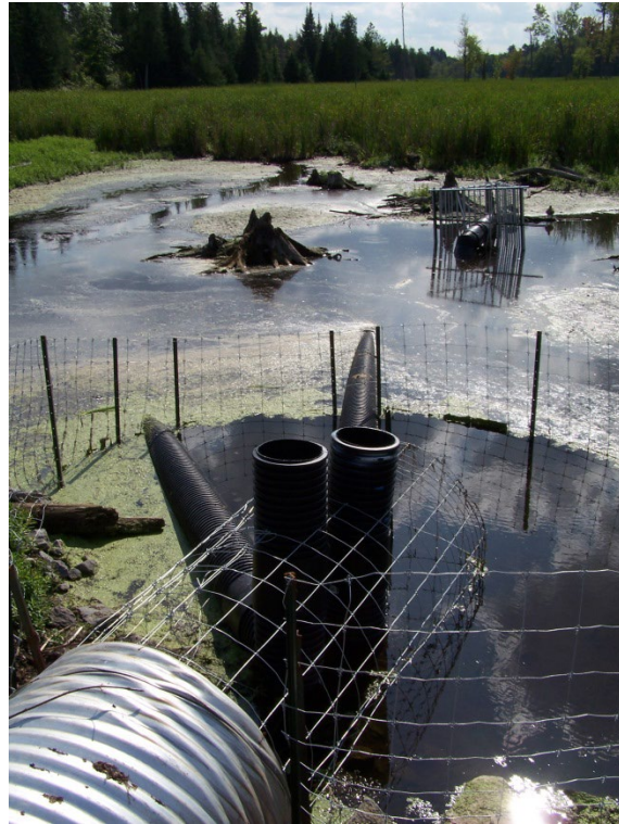
Figure 1. Goulbourn Forced Road Demonstration Site
