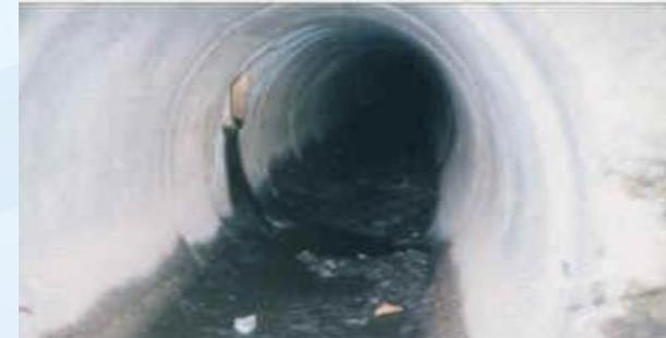
Wet weather conditions can result in sewer surcharge due to leaks in the pipe network as well as foundation and roof drain connections. This generates a risk of basement flooding.
