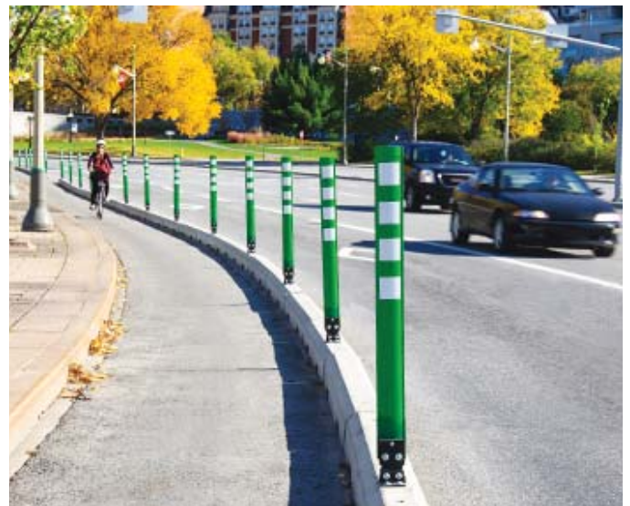
Figure 16: Flex-posts were discussed as a possible safety measure to combat increased traffic within the community. (Credit: Devlotech)
