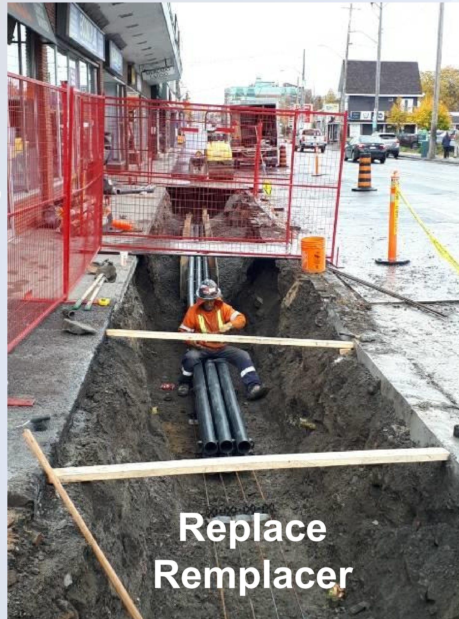
Hydro Ottawa work on Montreal Road - access to businesses maintained
