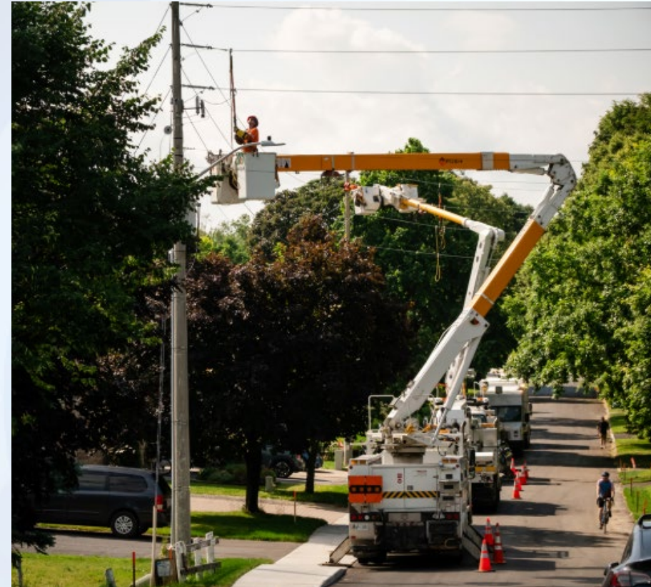
Typical construction image from HydroOttawa.ca ("Stay alert: You can keep our crews safe")
