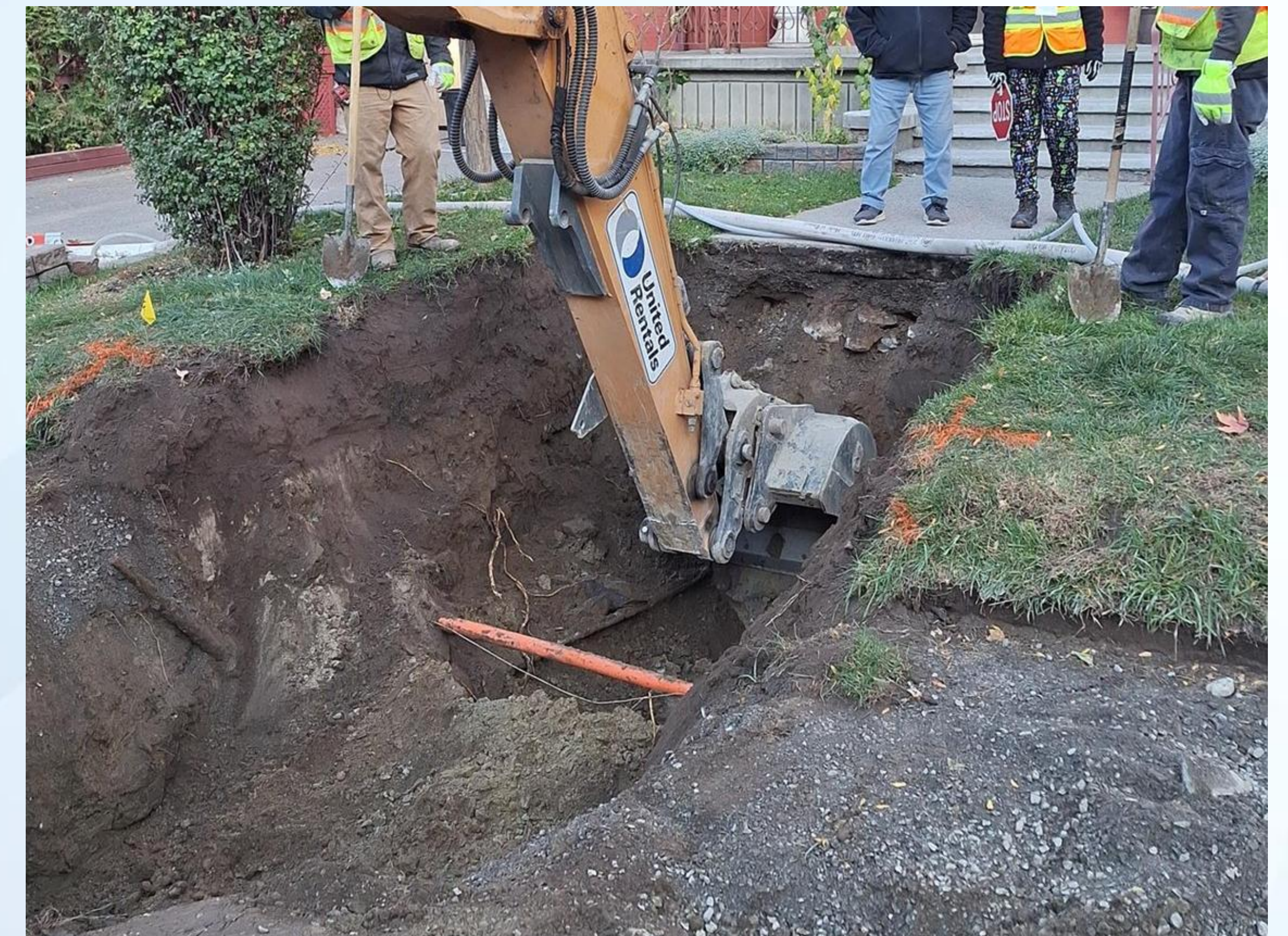
Service excavation up to property line
