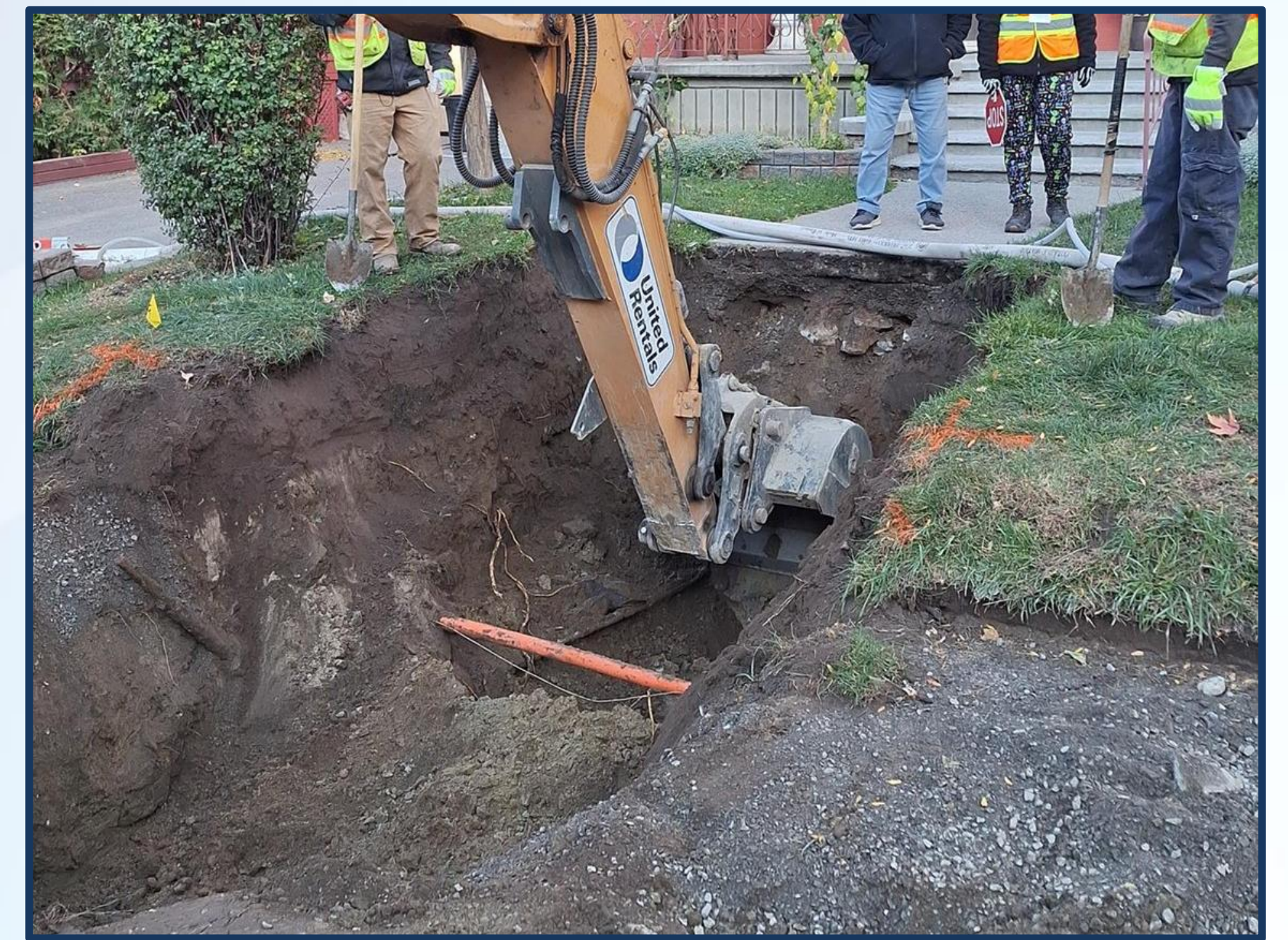
Service excavation up to property line
