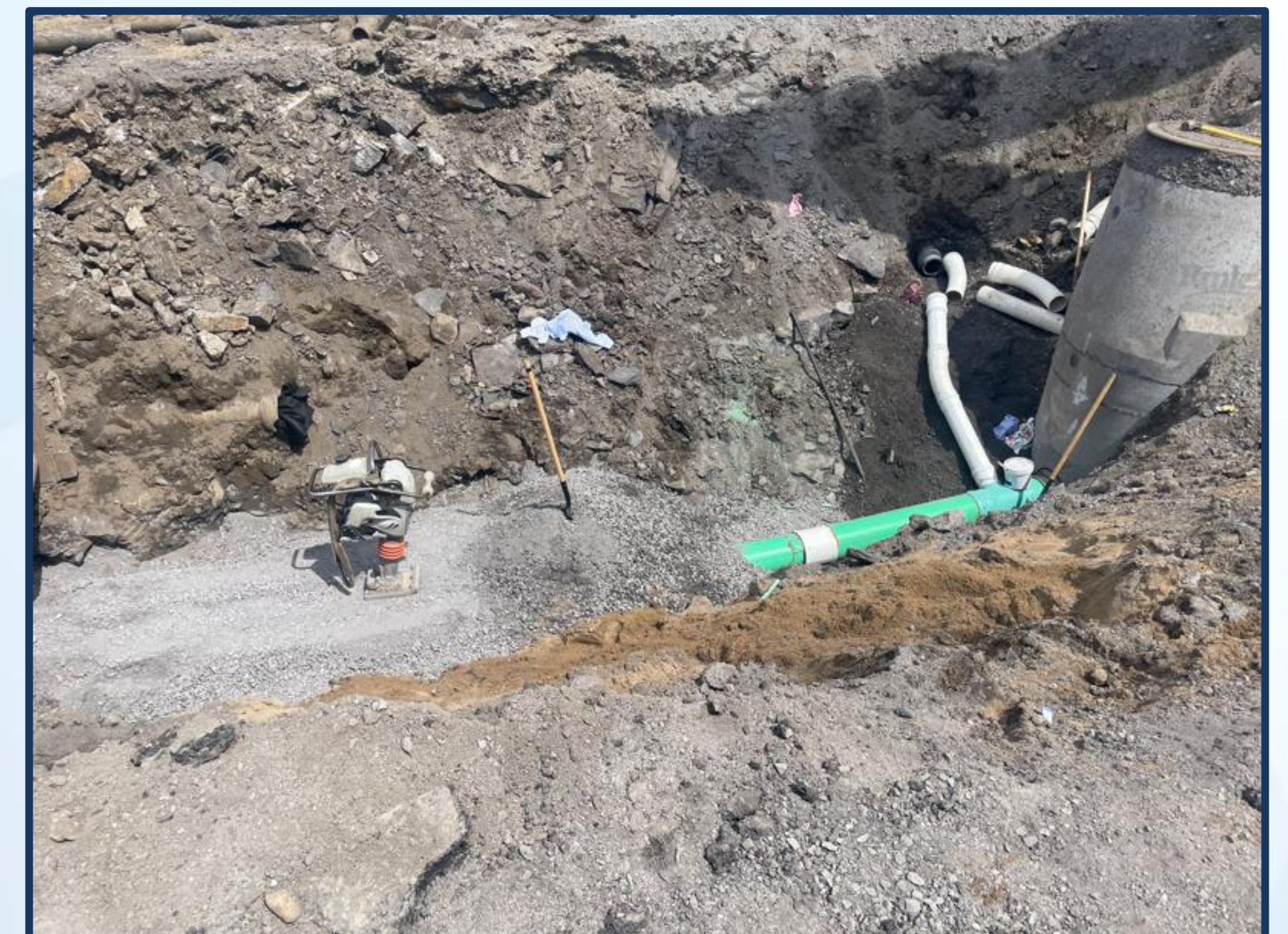
Typical water/sewer trench and installation
