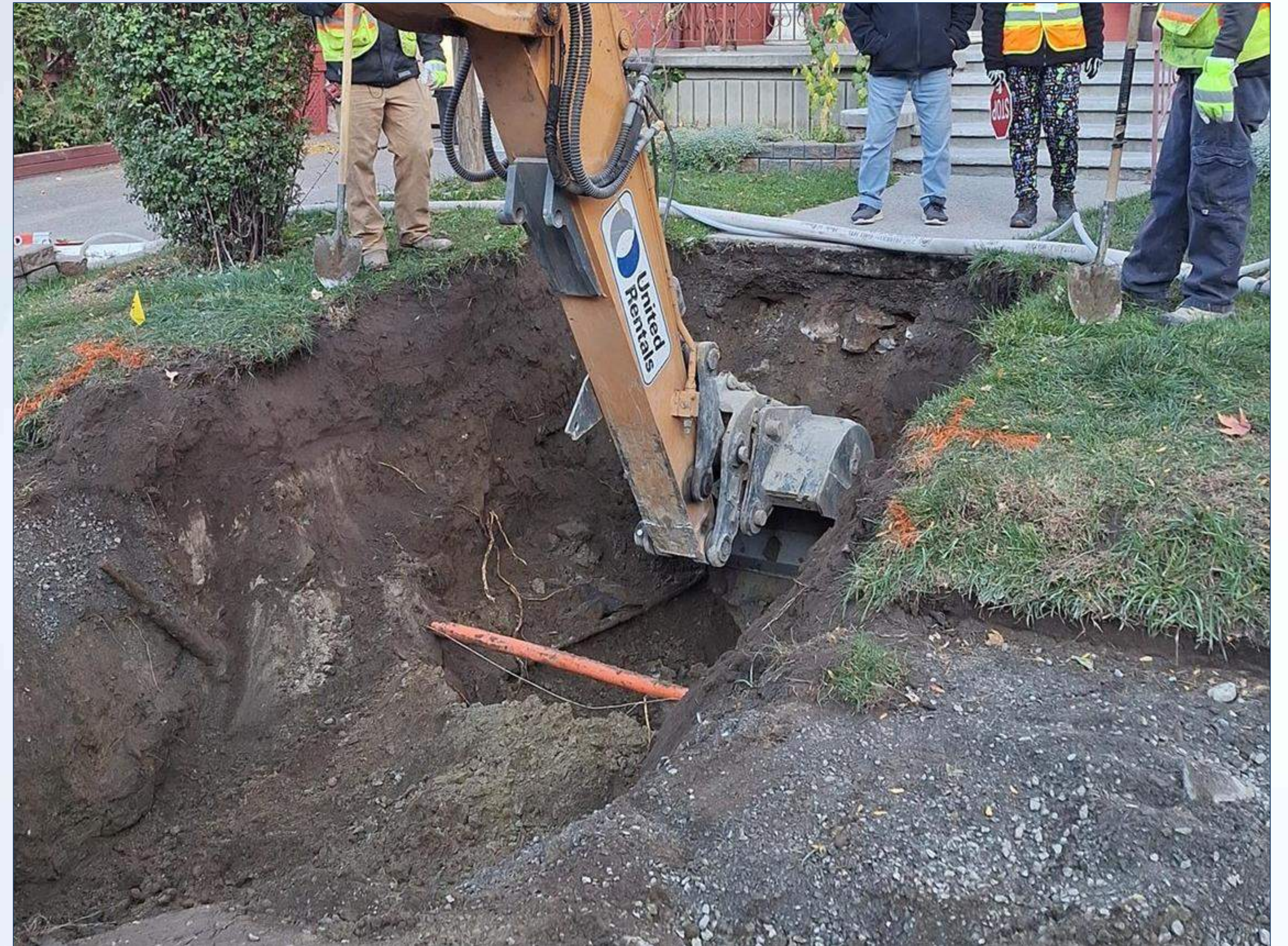
Service excavation up to property line
