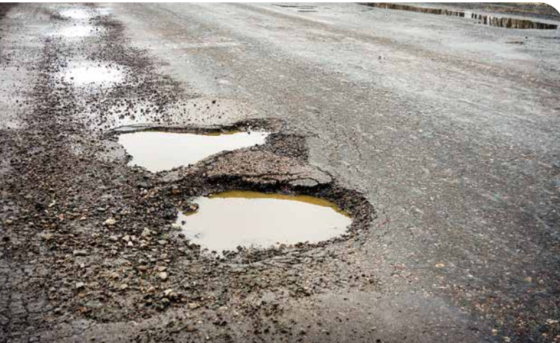
Image 16: Several potholes are seen on an asphalt road (left) and a newly installed rain garden (right)
