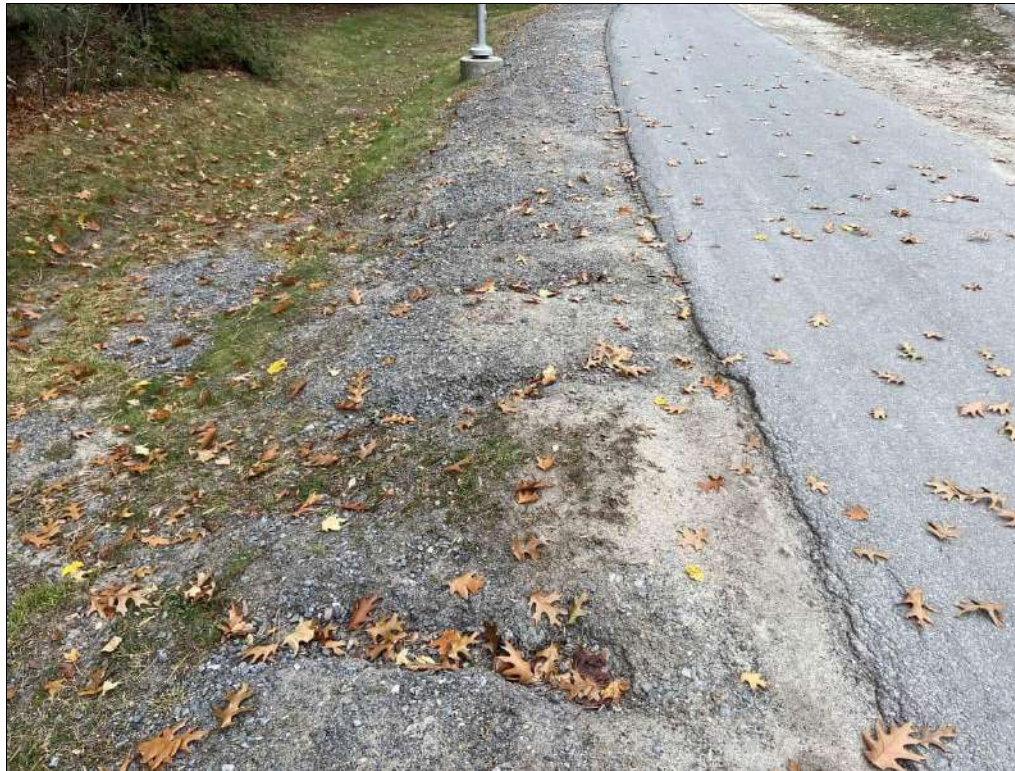
Photo 11: South Drainage Swale: General view of the swale. Road base material has eroded into the swale.
