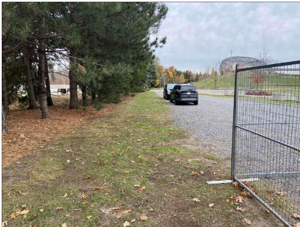
Photo 20: Former McElroy Building/Eastern Perimeter Drainage Swale: Areas of bare soil and stressed vegetation on either side of the gravel covered portion of this area.
