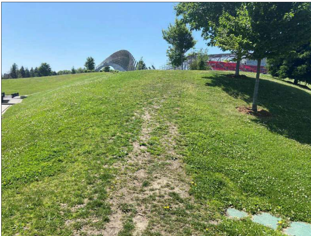
Photo 4: East Berm: Area of bare soil inferred to be from pedestrian traffic at the northwest end of the berm.
