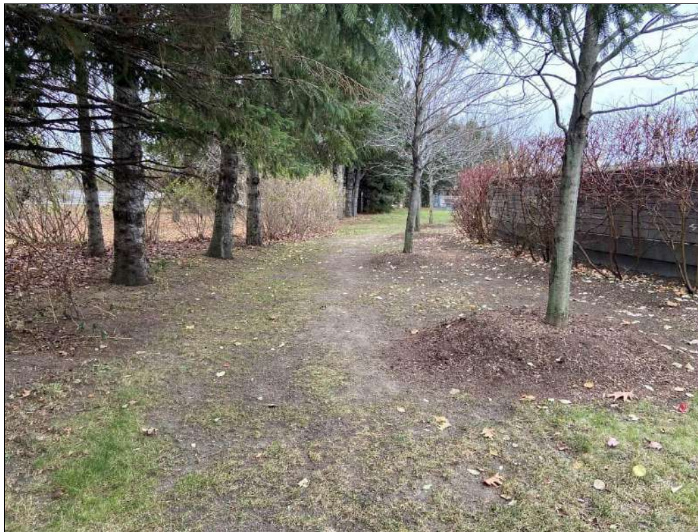
Photo 21: Eastern Perimeter Drainage Swale: Areas of bare soil and stressed vegetation east of the Water Plaza.
