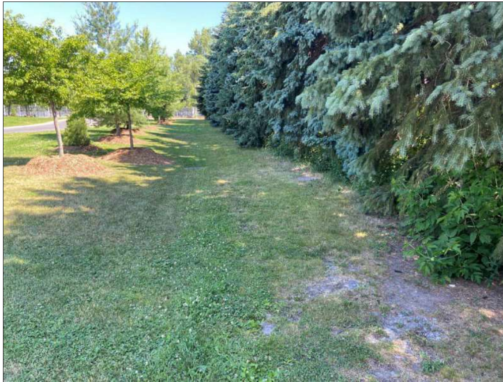
Photo 19: Eastern Perimeter Drainage Swale: General view of the swale east of the Ice Rink and Heirloom Orchard. Small areas of bare soil were observed in the area of the utility trench previously excavated within the swale.
