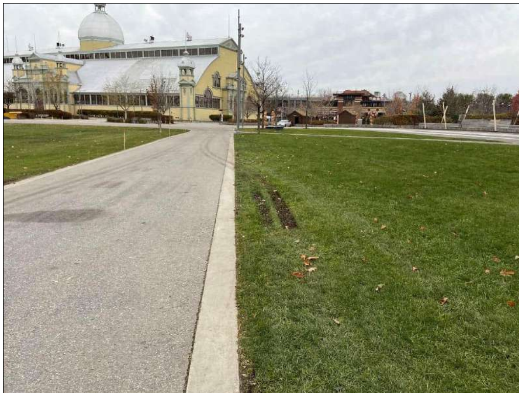
Photo 18: Former Eastern Landfill: Tire ruts were observed in the grassed area north of the Ring Road south of the Water Jet Plaza.
