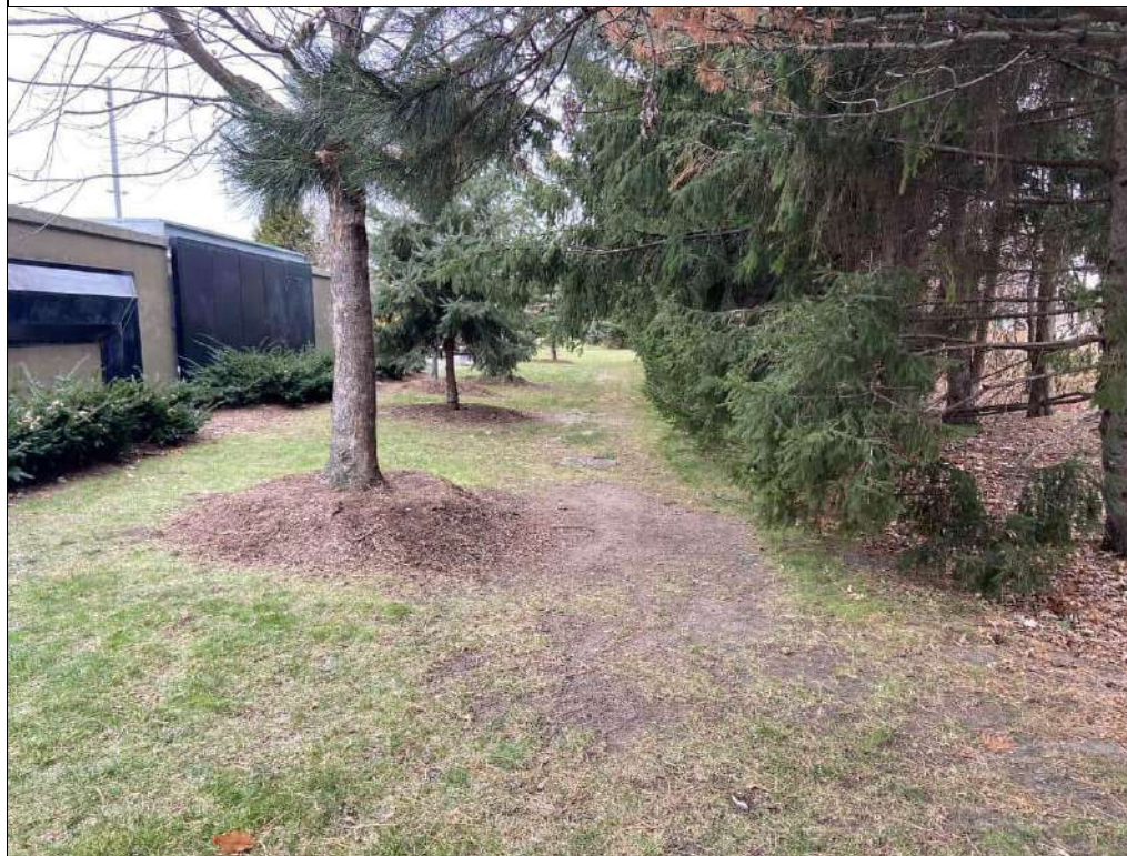
Photo 22: Eastern Perimeter Drainage Swale: Areas of bare soil and stressed vegetation east of the Childrens Garden.
