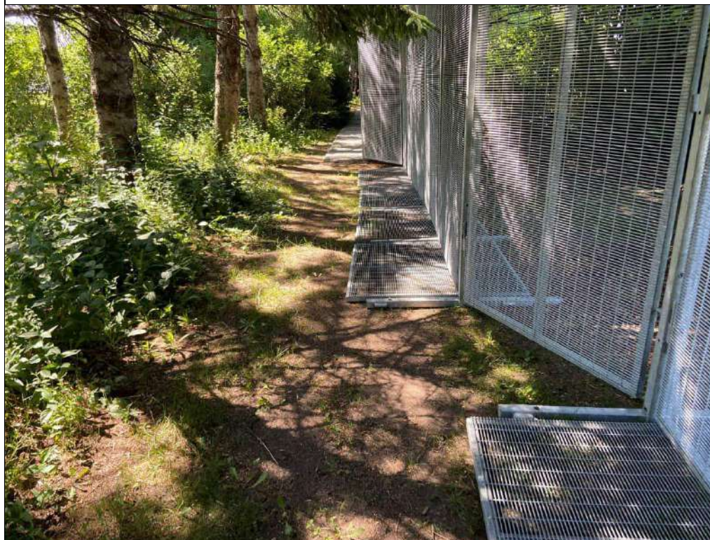
Photo 18: Eastern Perimeter Drainage Swale: Areas of bare soil and stressed vegetation east of the Water Plaza. Most of the area was being used as a staging area for the Escapade Music Festival.
