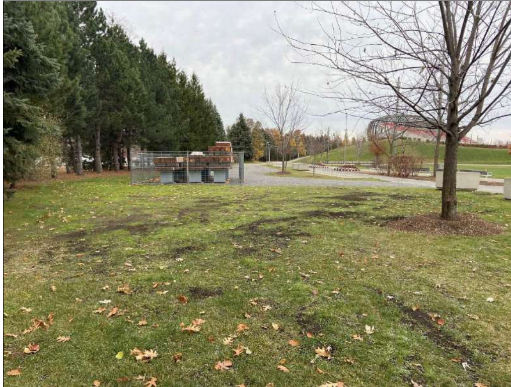
Photo 19: Eastern Perimeter Drainage Swale: The area east of the Water Jet Plaza is being rehabilitated. New topsoil and grass growing in this area.
