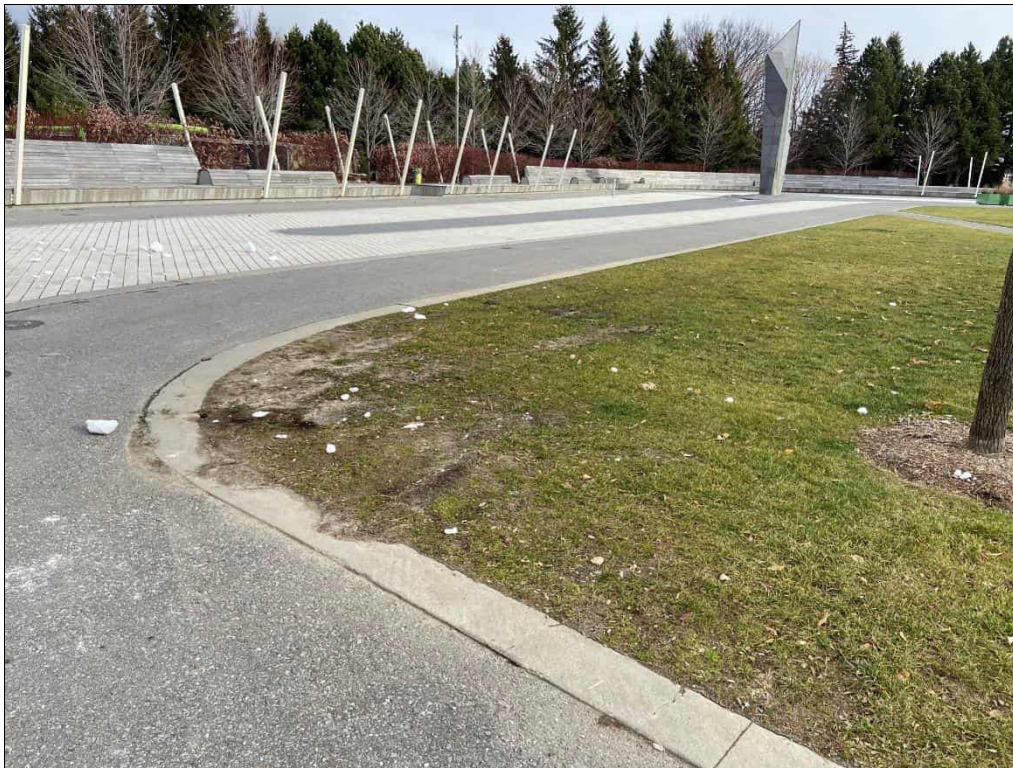
Photo 16: Former Eastern Landfill: Areas of bare soil were observed south of the water plaza.
