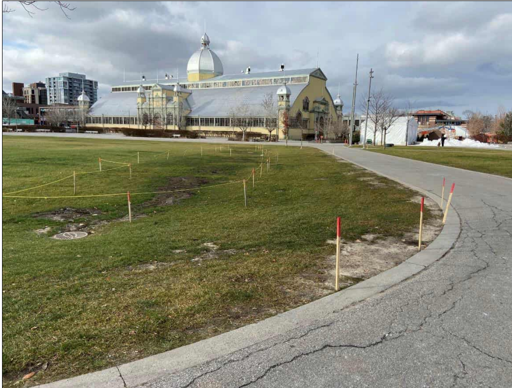
Photo 17: Former Eastern Landfill: Stressed vegetation and areas of bare soil were observed at the northeast end of the Great Lawn.
