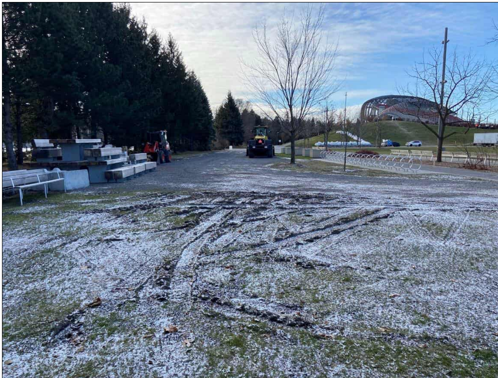
Photo 20: Eastern Perimeter Drainage Swale: Areas of bare soil and tire ruts were observed east of the Water Jet Plaza.
