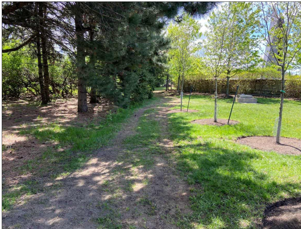
Photo 21: Eastern Perimeter Drainage Swale: Areas of bare soil and stressed vegetation east of the Water Plaza. Note: worn vehicular path.
