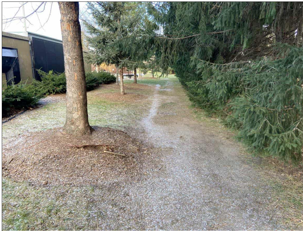
Photo 23: Eastern Perimeter Drainage Swale: Areas of bare soil and stressed vegetation east of the Children's Garden.
