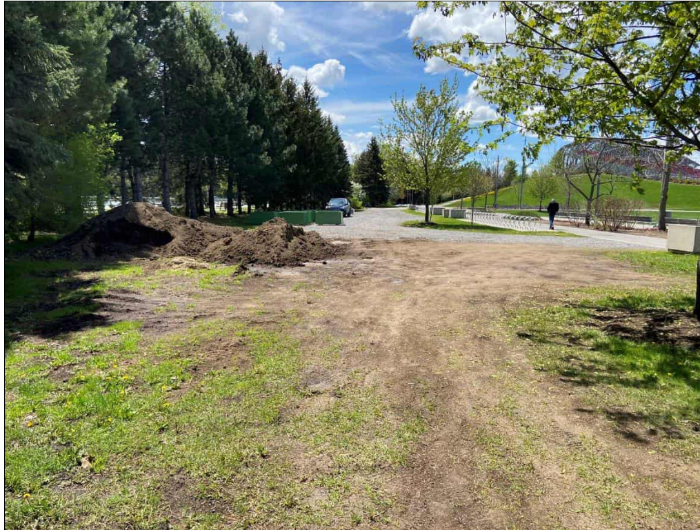
Photo 19: Eastern Perimeter Drainage Swale: Areas of bare soil and stockpiled topsoil were observed east of the Water Jet Plaza.
