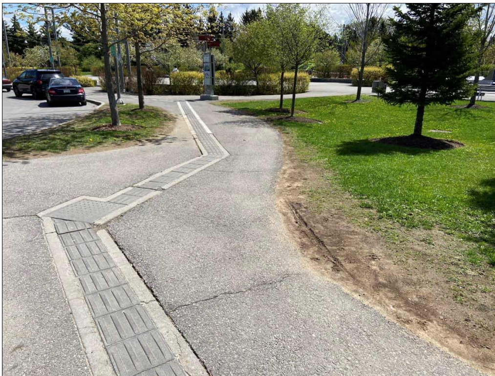
Photo 12: Former Eastern Landfill: Small areas of bare soil along pathways at the north end of the former landfill around the Skating Court.
