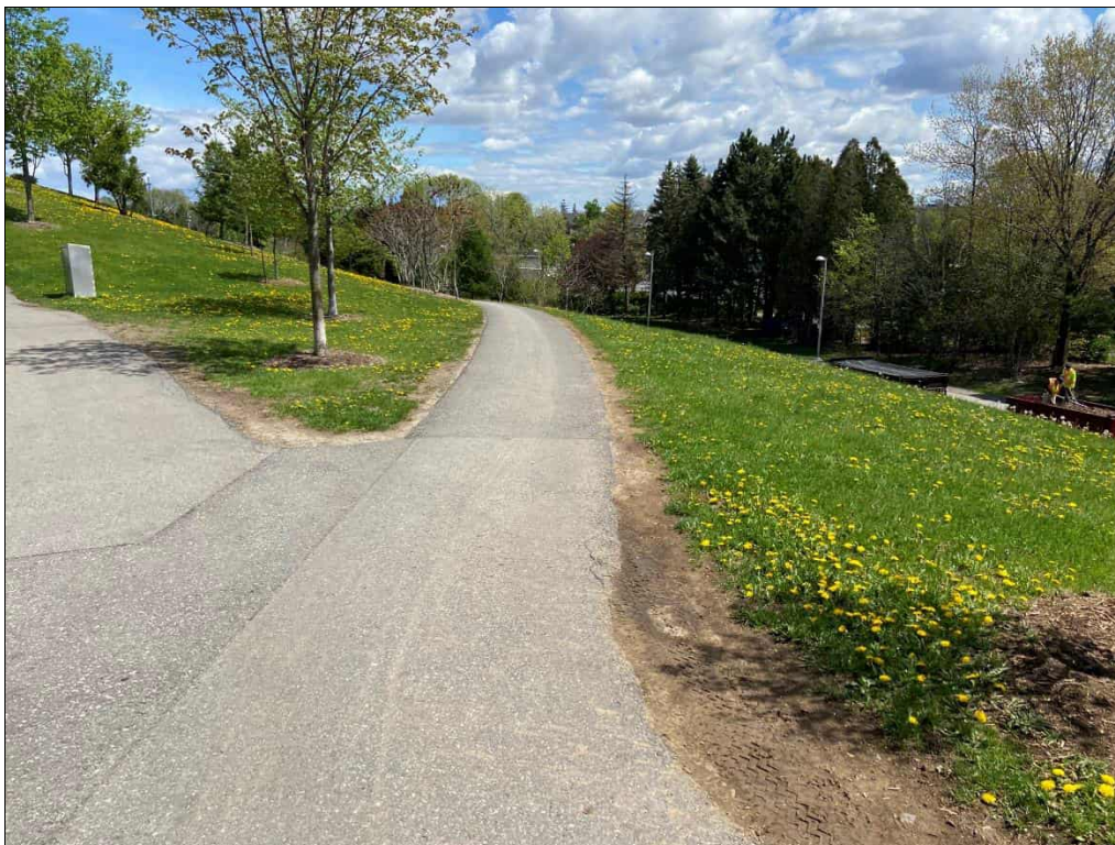
Photo 6: East Berm: Stressed vegetation and bare soil observed along the pedestrian pathway on the south side of the berm.
