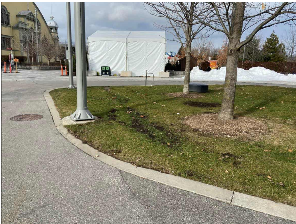
Photo 18: Former Eastern Landfill: Areas of bare soil were observed in the grassed area north of the Ring Road south of the Water Jet Plaza.
