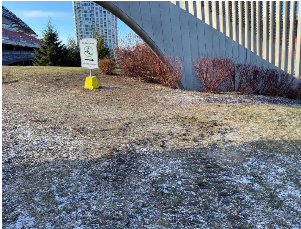
Photo 3: East Berm: Areas of bare soil were observed at the top of the berm.
