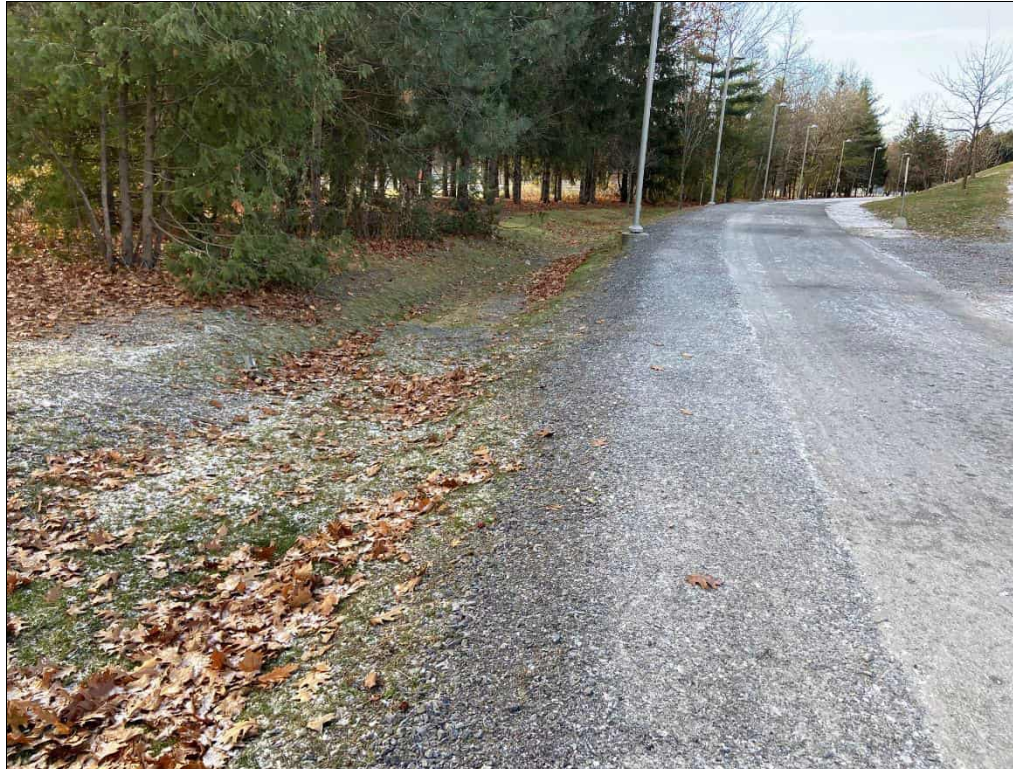
Photo 11: South Drainage Swale: General view of the swale. Road shoulder has been regraded.
