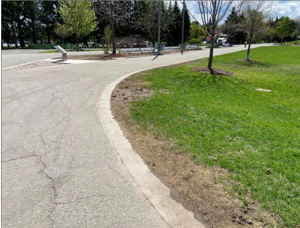
Photo 17: Former Eastern Landfill: Stressed vegetation and areas of bare soil were observed at the northeast end of the Great Lawn. Some of these areas had grass seed.
