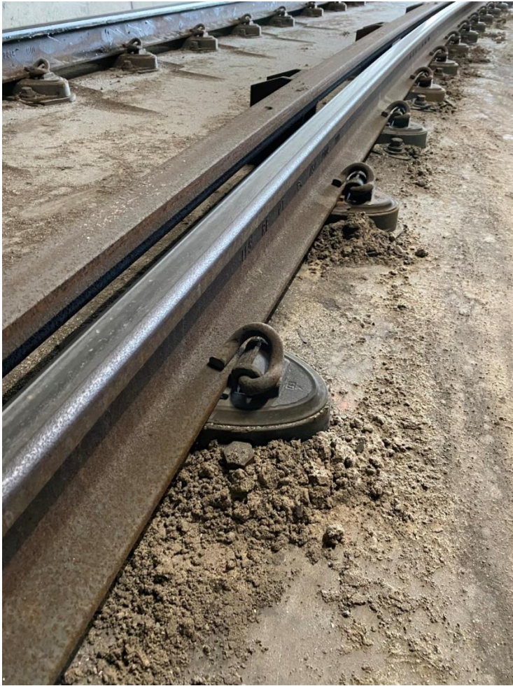
Figure 4.19: Sand accumulated at East Connector Due to Excessive Wheel Spin/Slide Caused by Presence of Grease on Top of Rail
