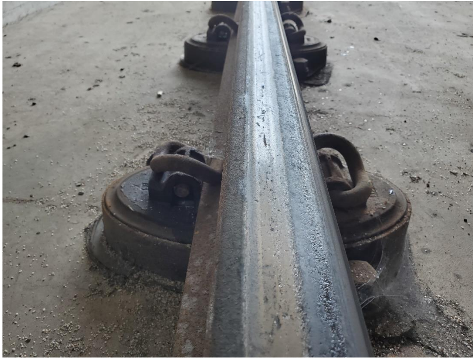
Figure 5.7: Grease on Rail Crown at Manual Grease Application Location
