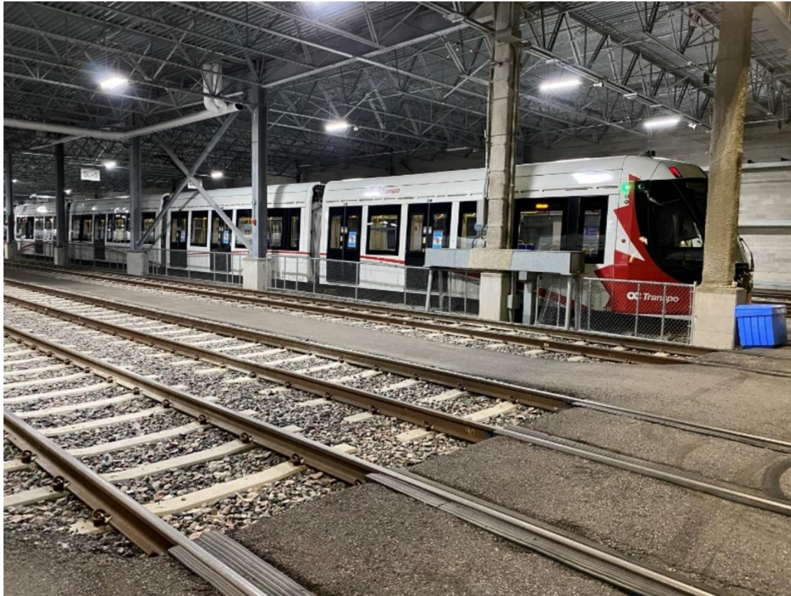
Figure 4.9: Dividing Fence at Storage Shed and Limited Staff Access Between Tracks with No Walkway
