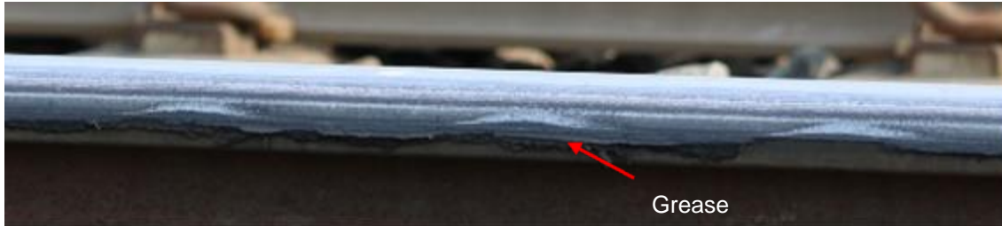
Figure 3.13: Corrugation on High Rail of Curve 230 at 105+655
