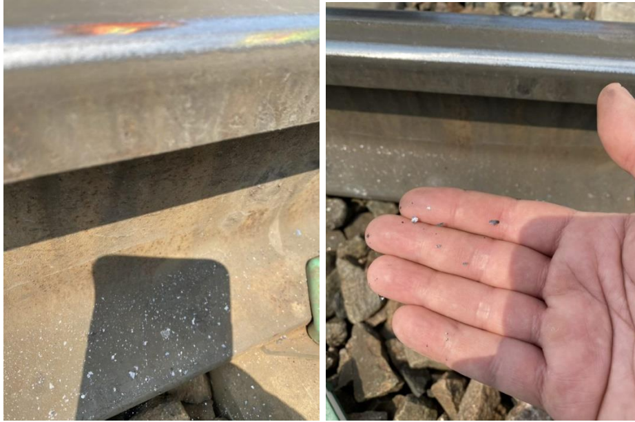
Figure 5.3 & 5.4: Metal Shavings at Curve 19
