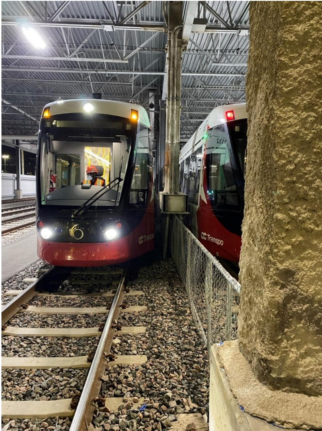
Figure 4.10: Dividing Fence at Storage Shed with No Staff Access or Safety Clearance
