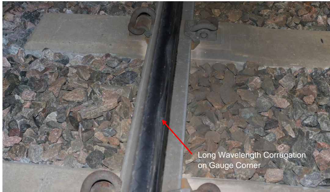
Figure 3.12: Corrugation on High Rail of Curve 330 at 108+685
