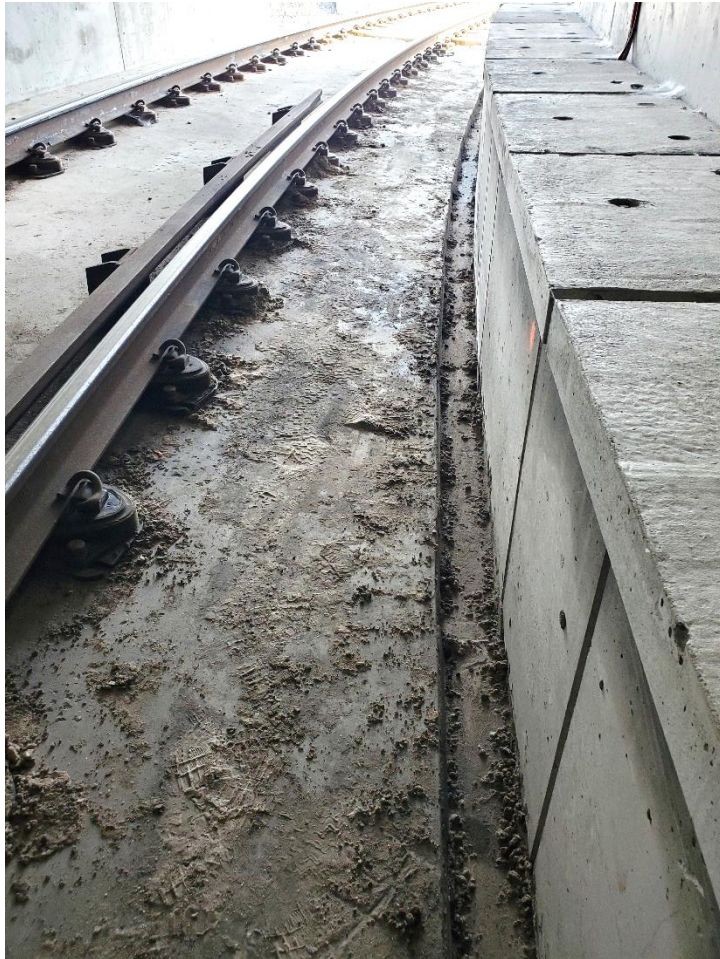
Figure 5.9: Sand in East Connector Portal Tunnel
