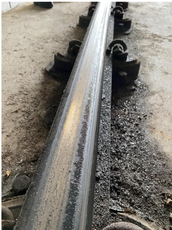
Figure 4.18: Grease on Top of Rail at East Connector
