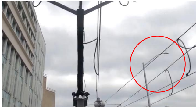
Figure 3.40: OCS to OCS at Crossovers and Turnouts
