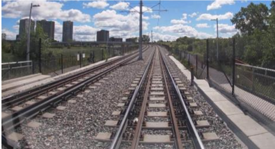
Figure 3.7: Expansion joints installed in a “facing” position on the eastbound line
