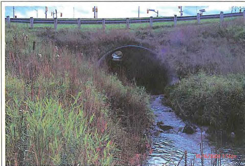
Photograph Description- North end. Photo # P0000052
