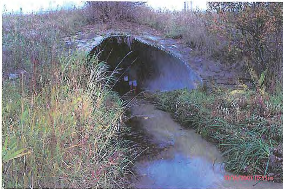
Photograph Description- South end. Photo #- P0000018
