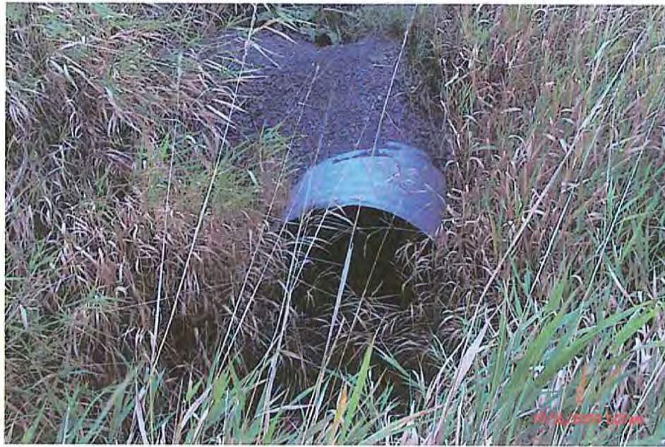
Photograph Description- South end. Photo #- P0000035
