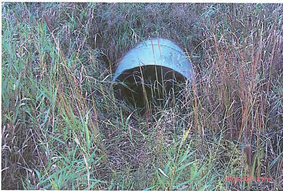
Photograph Description- North end. Photo #- P0000045
