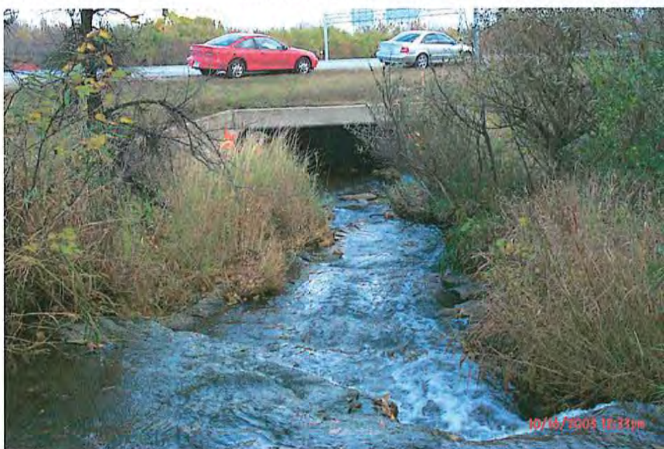
Photograph Description- South end. Photo #- P0000031
