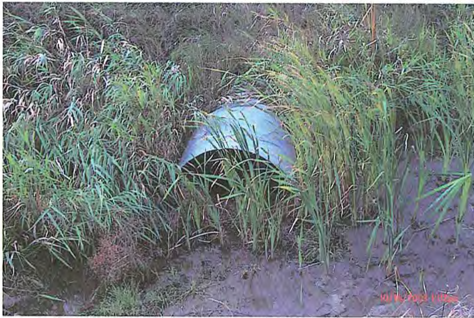
Photograph Description- North end. Photo #- P0000034
