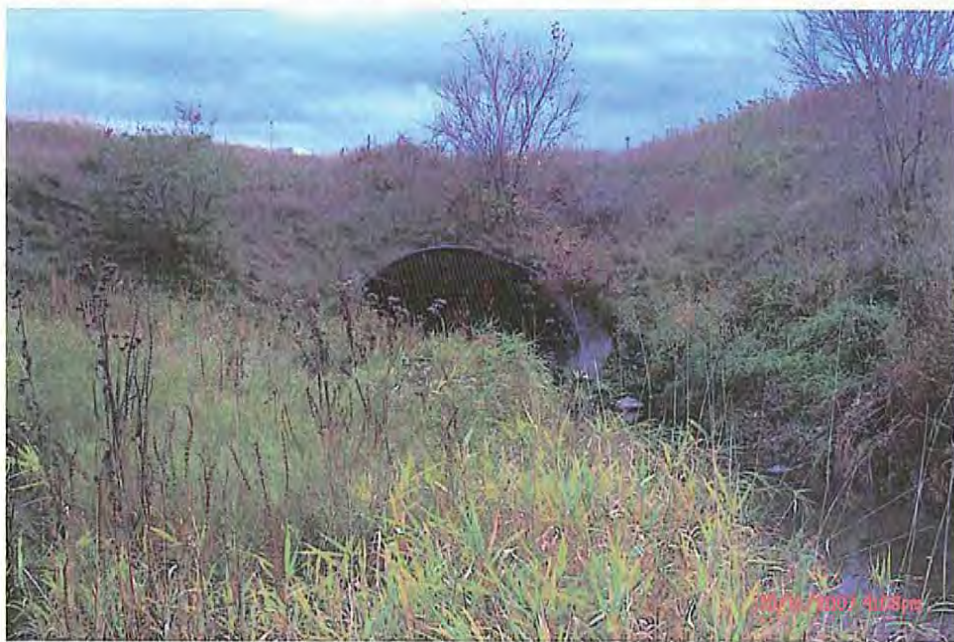
Photograph Description- North end. Photo #- P0000054
