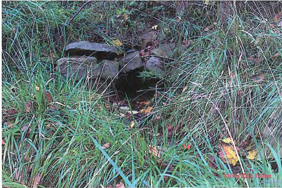
Photograph Description- North end. Photo #- P0000046
