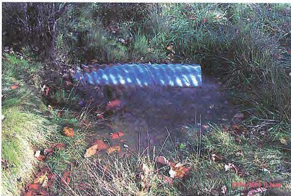
Photograph Description- South end. Photo #- P0000021
