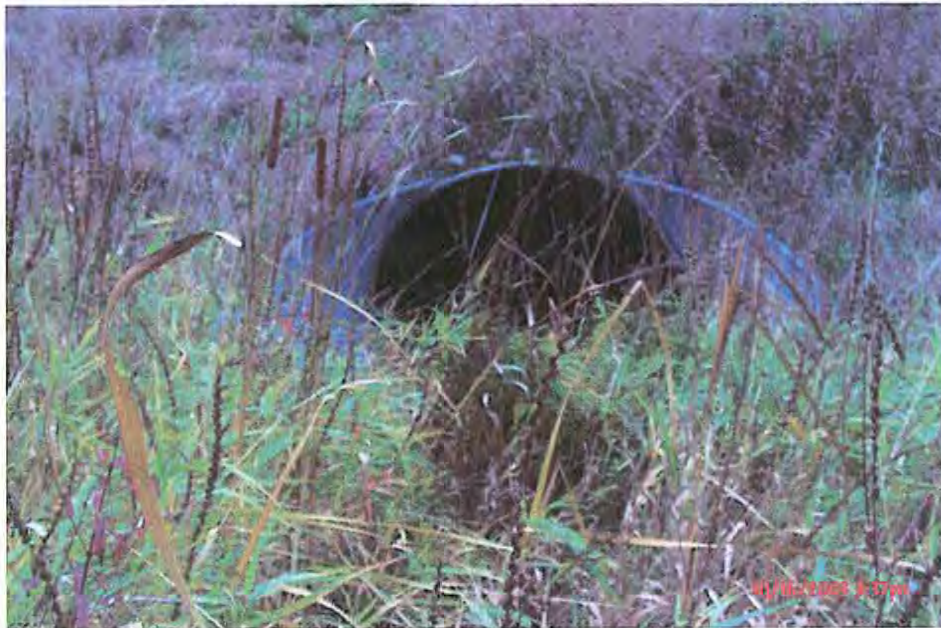
Photograph Description – South end. Photo # P0000049
