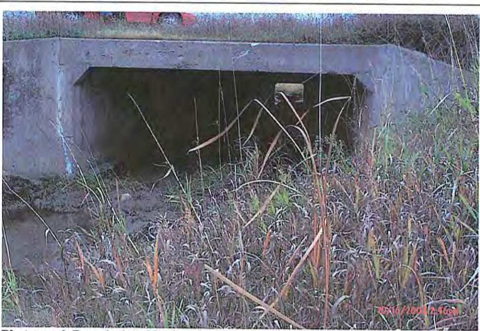
Photograph Description- North end. Photo #- P0000044
