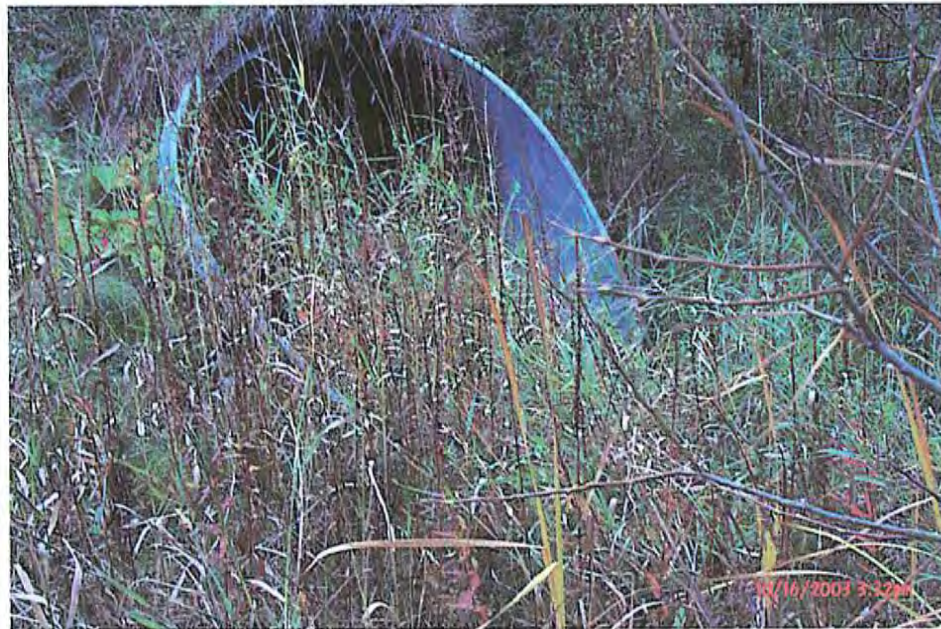
Photograph Description- North end. Photo # P0000048
