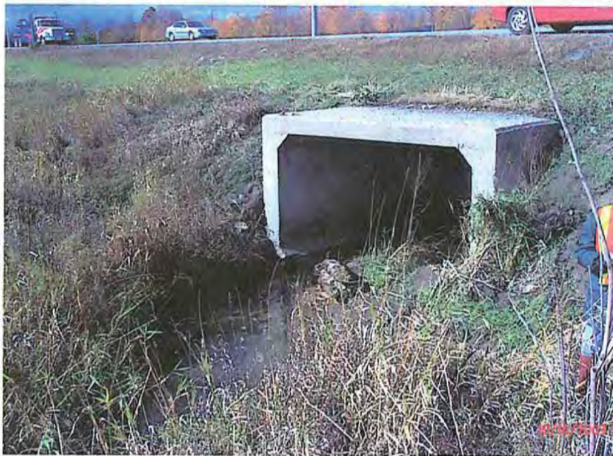
Photograph Description- South end. Photo #- P0000033
