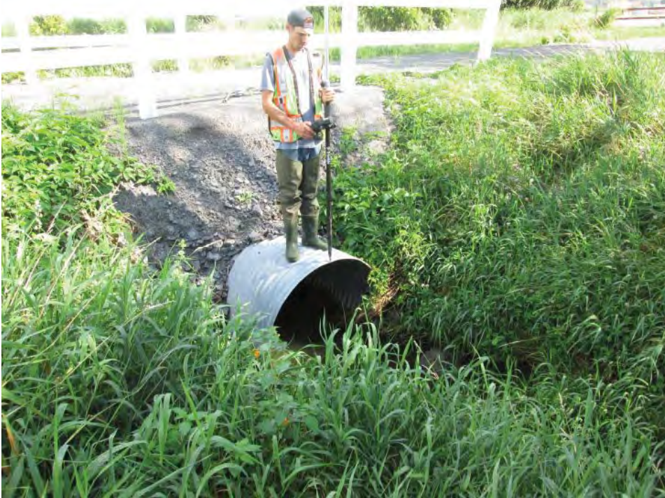
Photograph 12 Looking upstream (south) at the downstream face of the 1200 mm corrugated metal pipe under the Wesley Clover Farms path
