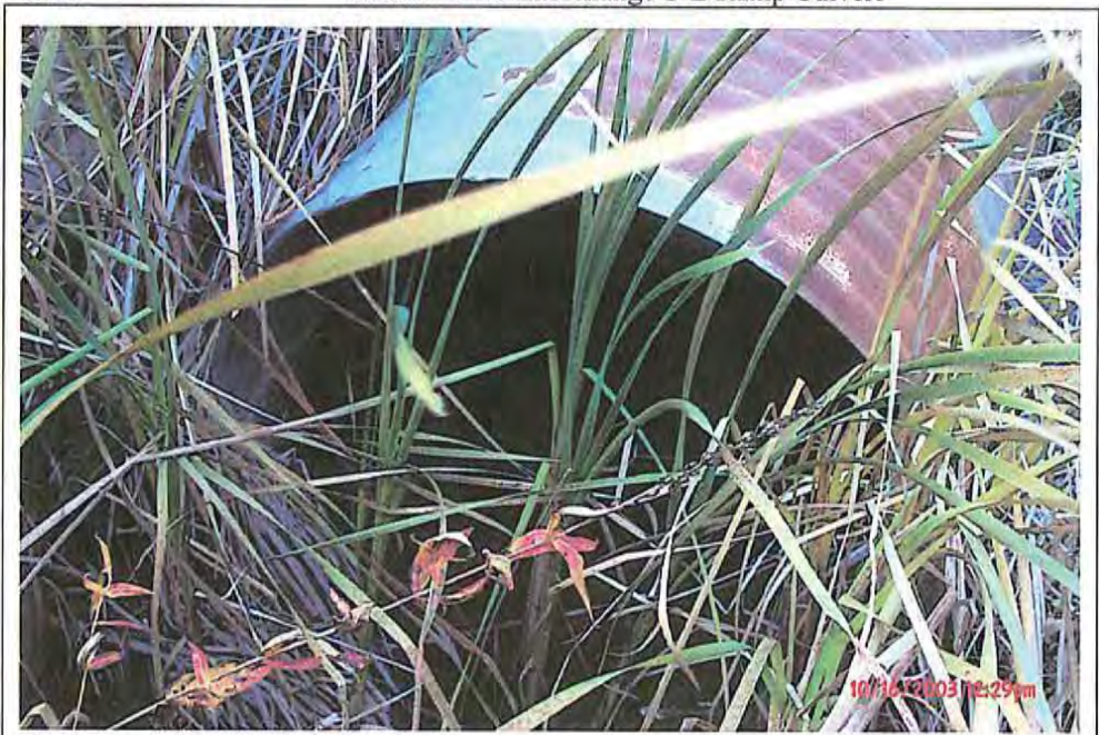
Photograph Description- South end. Photo #- P0000030
