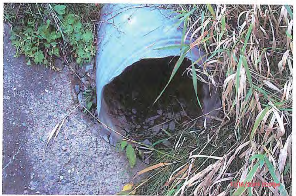
Photograph Description- South end. Photo #- P0000025
