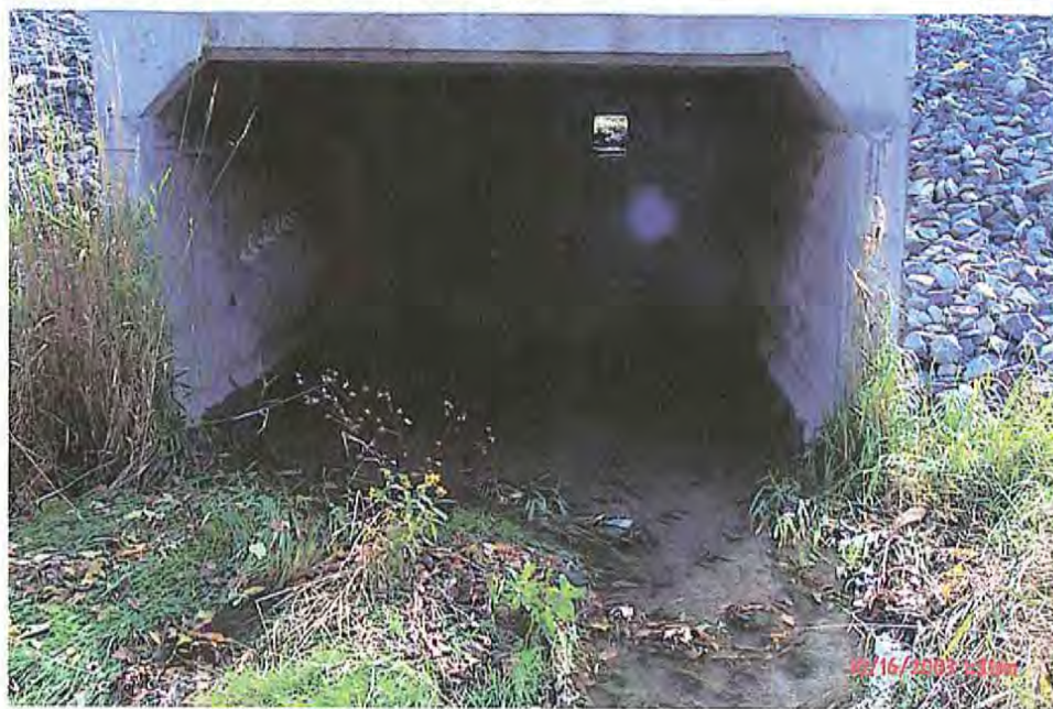
Photograph Description- North end. Photo #- P0000037
