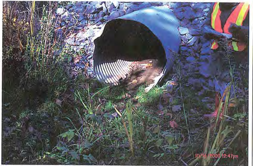
Photograph Description- South end. Photo #- P0000032
