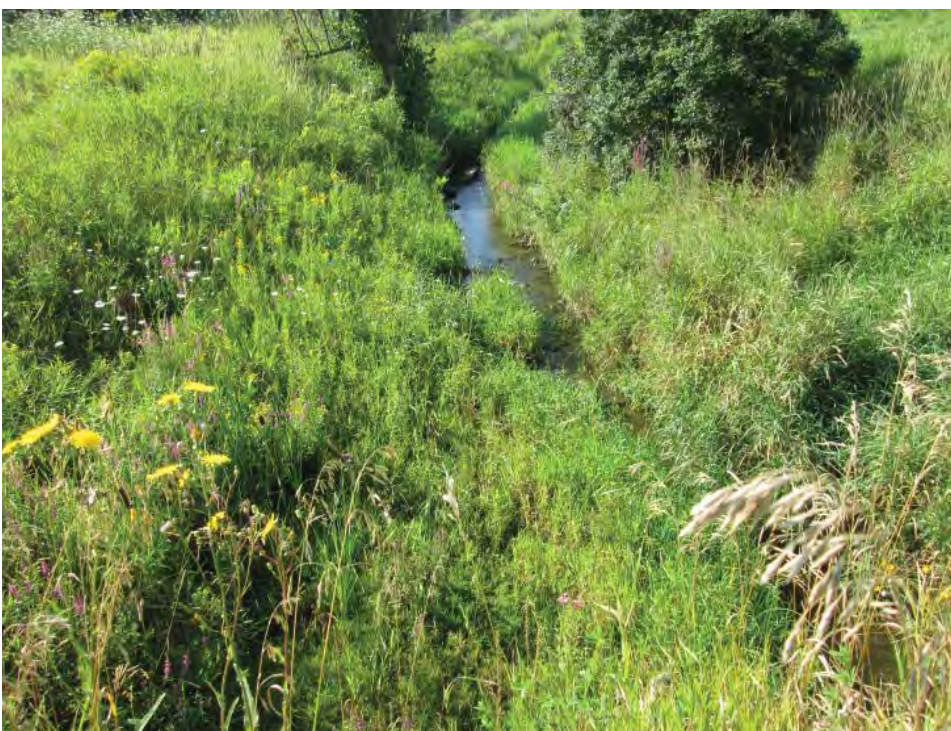
Photograph 11 Looking downstream (north) from the Corkstown Road 3.0 meter span by 2.0 meter rise open bottom box culvert
