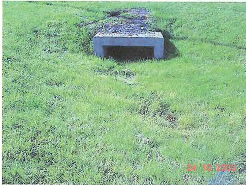
Photograph Description – East end. Photo # Mvc-259s
