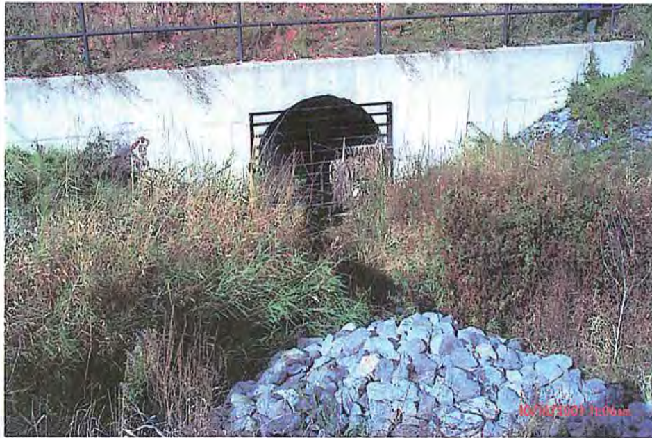
Photograph Description- South end. Photo #- P0000019
