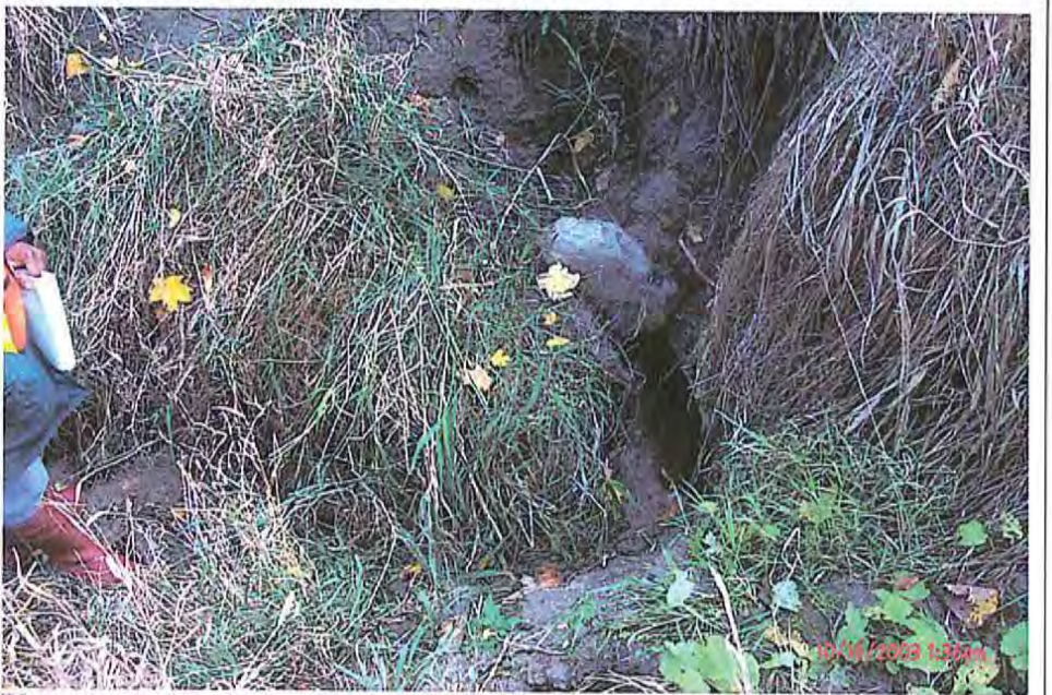
Photograph Description- North end. Photo #- P0000038
