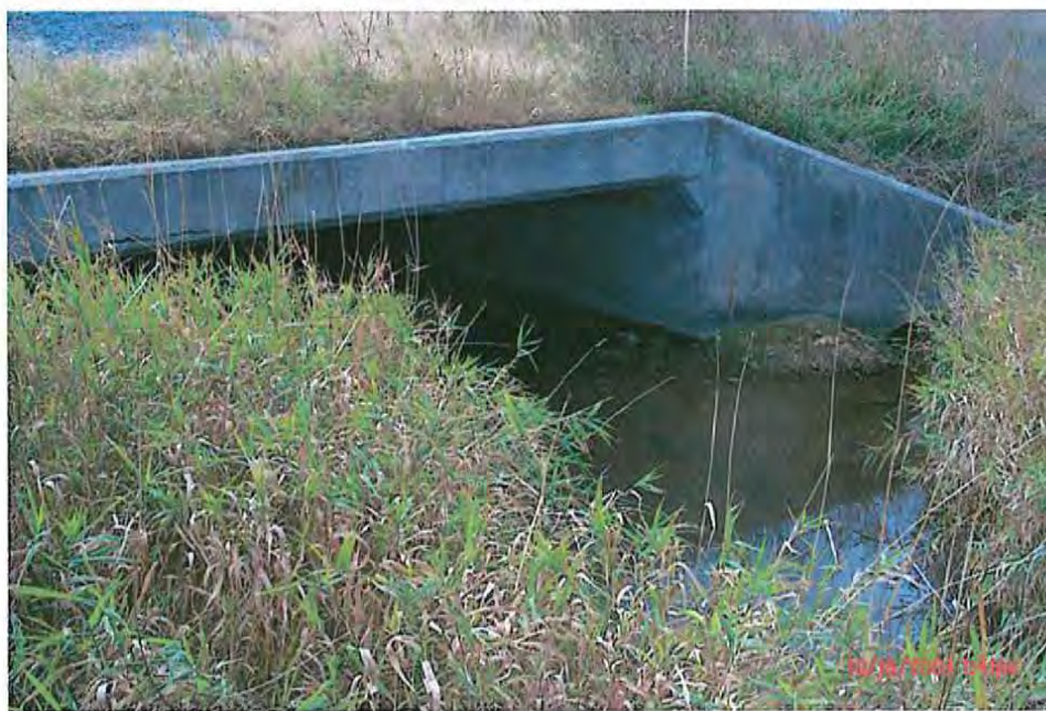
Photograph Description- North end. Photo #- P0000039
