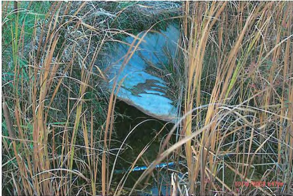
Photograph Description- South end. Photo #- P0000041
