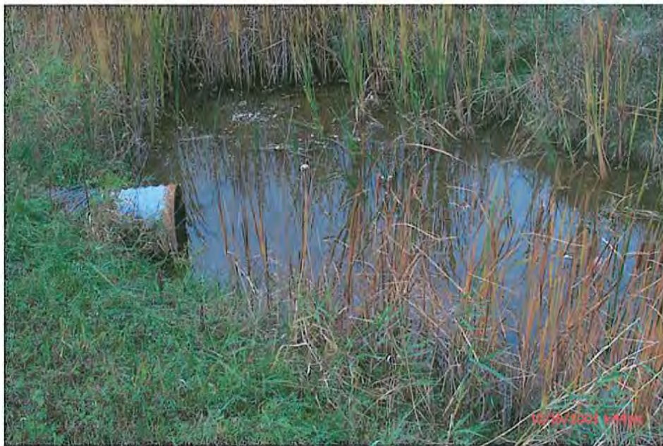
Photograph Description- North end. Photo #- P0000040
