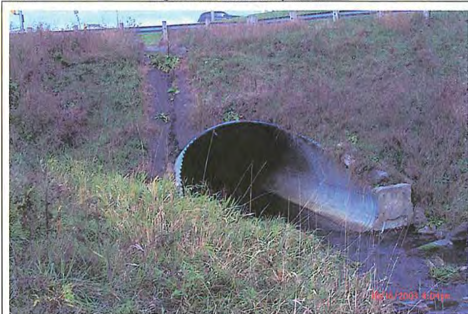
Photograph Description – South end. Photo # P0000053
