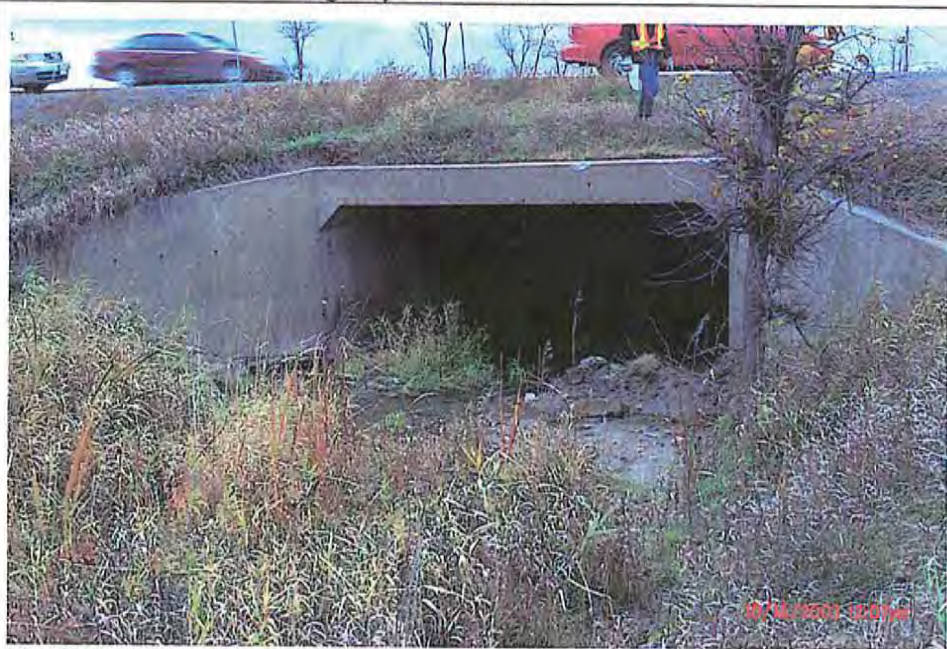
Photograph Description- South end. Photo #- P0000026
