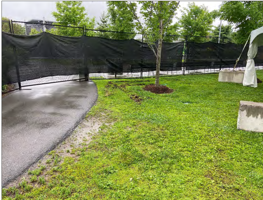
Photo 15: Former Eastern Landfill: Small areas of bare soil and stressed vegetation were observed in high traffic areas around the Skate Park and Children's Garden.
