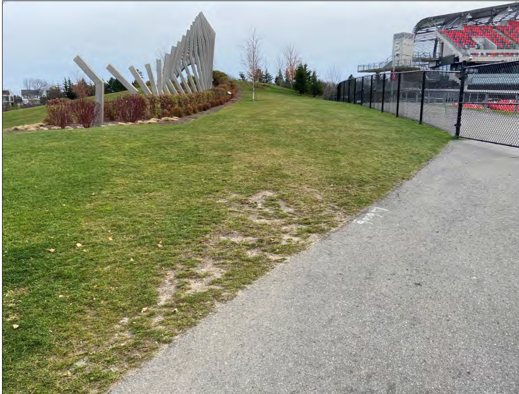
Photo 5: East Berm: Areas of bare soil west of the Art Screen near the pedestrian pathway.
