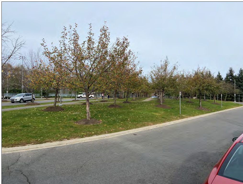
Photo 12: Former Eastern Landfill: Cover in the Orchard area along the roadway repaired in the Spring.
