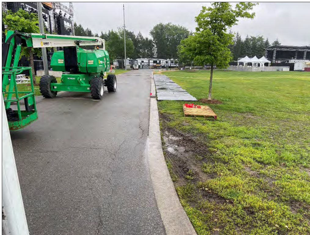
Photo 16: Former Eastern Landfill: Areas of bare soil and stressed vegetation south of the ring road at the north end the Great Lawn. Tire ruts were observed in this area and it was partially covered in preparation for the Escapade Music Festival.
