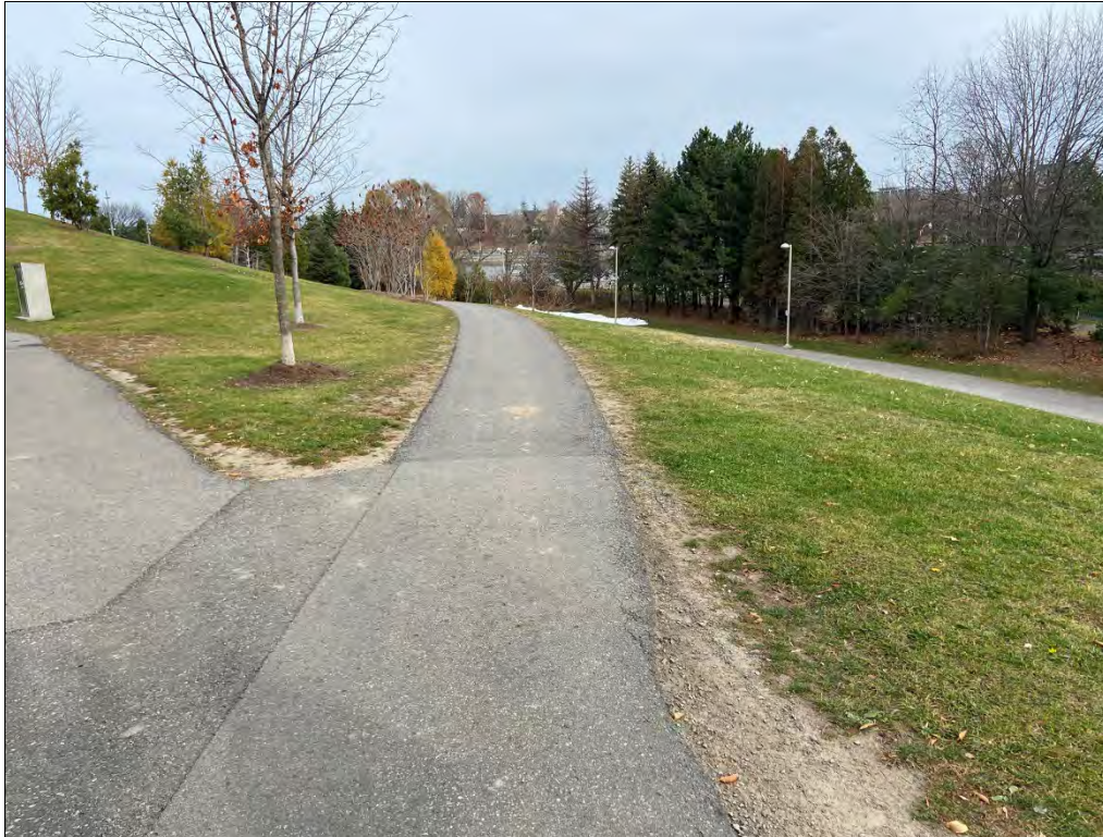
Photo 9: South Berm: Areas of bare soil along paths on the berm.
