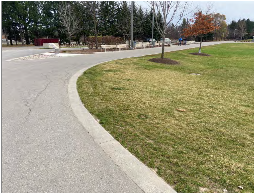
Photo 15: Former Eastern Landfill: Soil cover at the northeast east of the Great Lawn repaired in the Spring.
