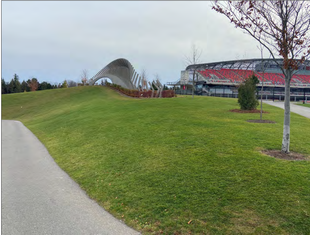
Photo 1: East Berm: General view of the east side of the berm.
