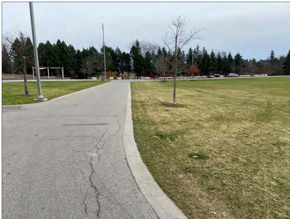
Photo 16: Former Eastern Landfill: Areas of stressed vegetation south of the ring road at the north end of the Great Lawn.
