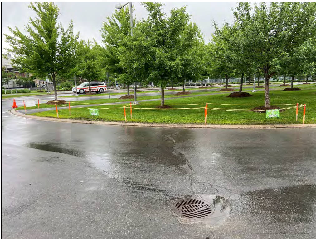
Photo 14: Former Eastern Landfill: Damaged areas of the cover in the Orchard were repaired.
