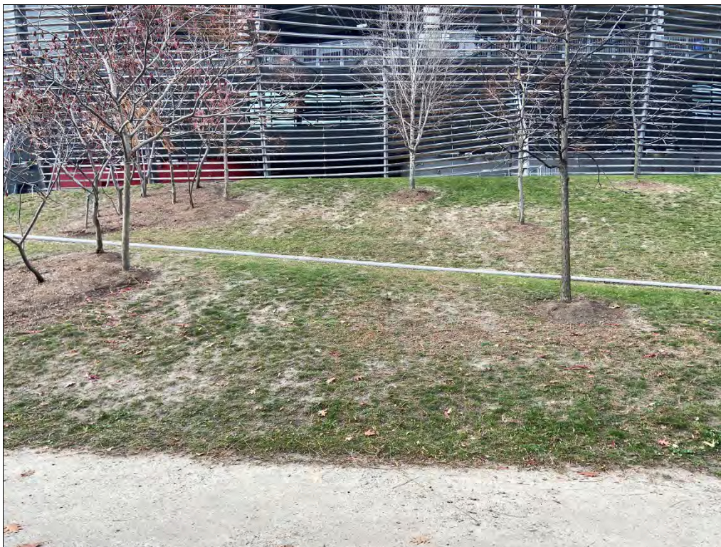
Photo 6: South Berm: General view of berm conditions. Areas of bare soil were observed throughout the berm.
