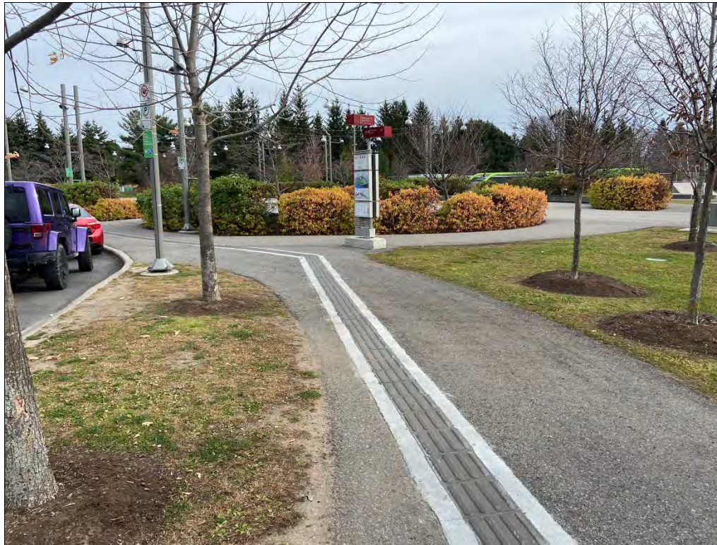
Photo 11: Former Eastern Landfill: Bare soil along pathways and roadways at the north end of the former landfill west of the Orchard.
