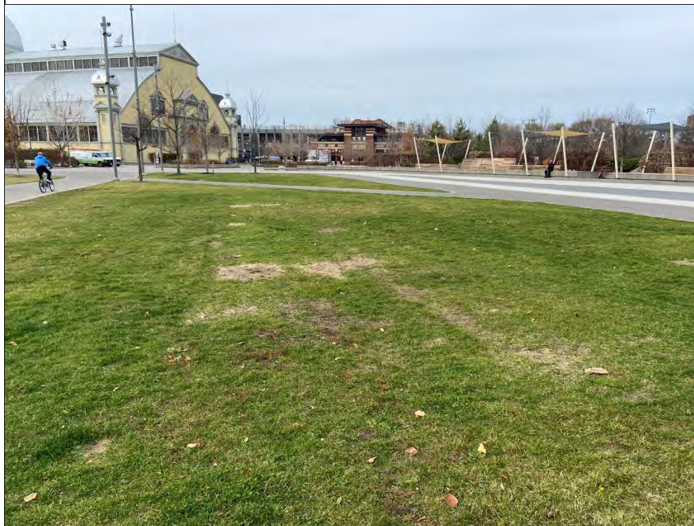
Photo 16: Former Eastern Landfill: Stressed vegetation and areas of bare soil where infrastructure for events is routinely erected south of the Water Plaza.
