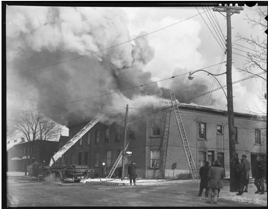
Figure 6: Fire, apartment house at Hill and Wellington St., 1955, City of Ottawa Archives | CA031295
