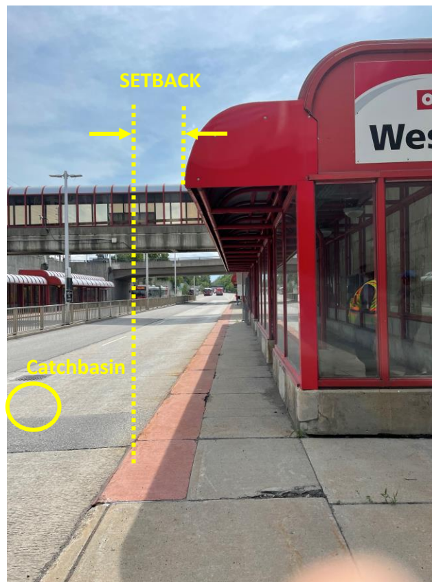
FIGURE 4: Westboro Station Canopy
