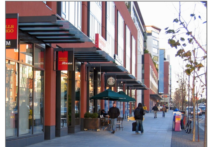
Figure 54: Ground-floor retail with awnings and high floor-to-ceiling measurements
