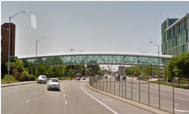
Figure 3-13 Pedestrian bridge across Woodroffe Avenue looking south
