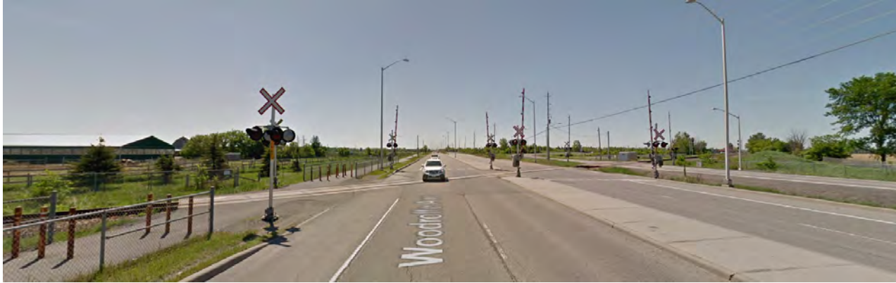
Figure 3-26 Woodroffe Avenue VIA Rail line at-grade crossing looking south. Southwest Transitway crossing (west) and MUP crossing (east)
