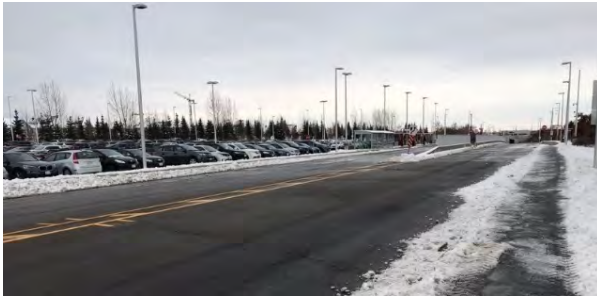
Figure 3-31 MUP located to the east of the Southwest Transitway underpass at Highbury Park looking south
