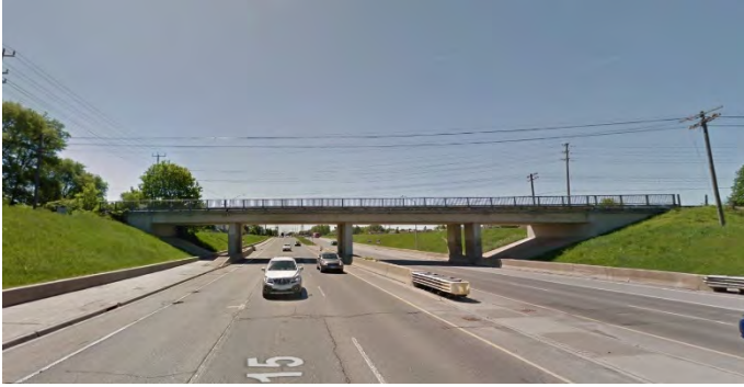
Figure 3-18 CN Rail line overpass of Woodroffe Avenue
