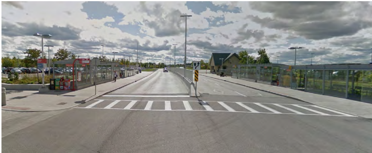
Figure 3-27 Fallowfield Transit Station on the Southwest Transitway looking west. VIA Rail Station (west)
