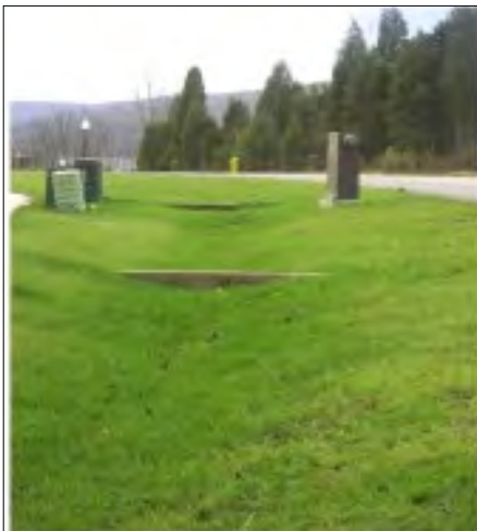
Figure 7-11 Enhanced Grass Swale with Check Dams (TRCA, 2016)
