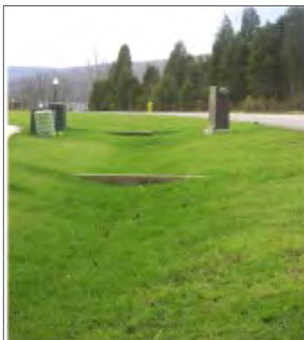
Figure 7-11 Enhanced Grass Swale with Check Dams (TRCA, 2016)
