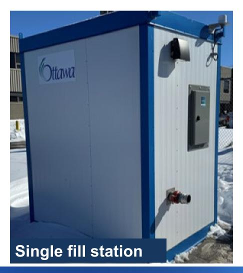
Installation of a backflow prevention device is not required when using the bulk fill station as one is permanently installed in the station itself.
