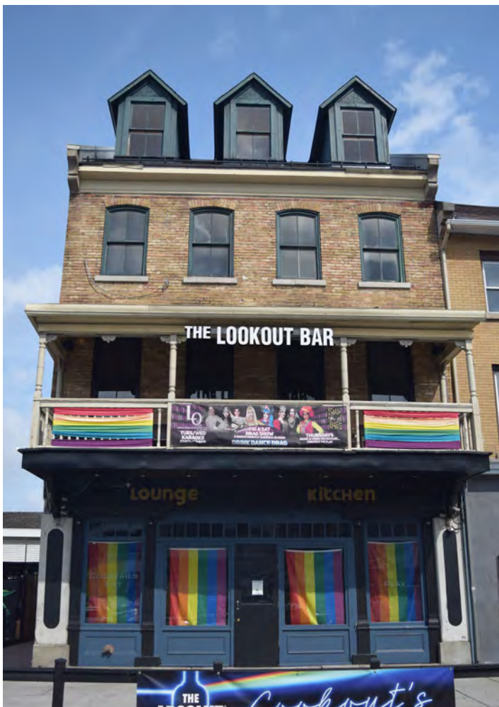
Figure 37: 41 York street with its sloped roof and dormers.
