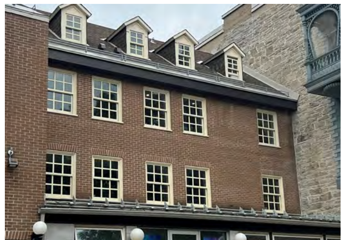
Figure 45: Dormers in Sussex Courtyards.
