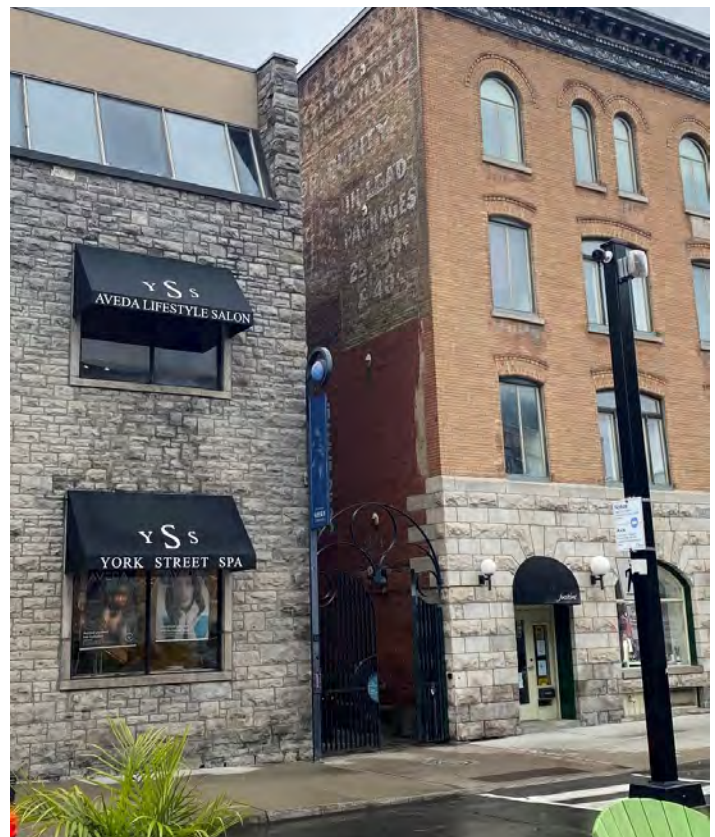
Figure 31: Two buildings on York Street with current awning signs and remnants of a former painted ghost sign.
