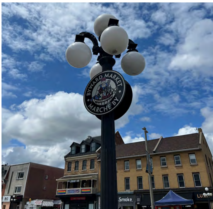
Figure 57: Example of the revamped five globe street light in the market.
