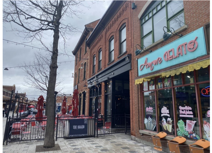
Figure 3: Mixed use buildings at William Street mall.
