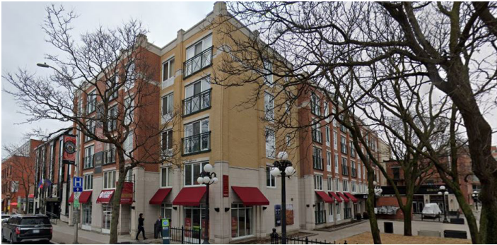
Figure 48: Example of compatible new construction facing Murray Street.
