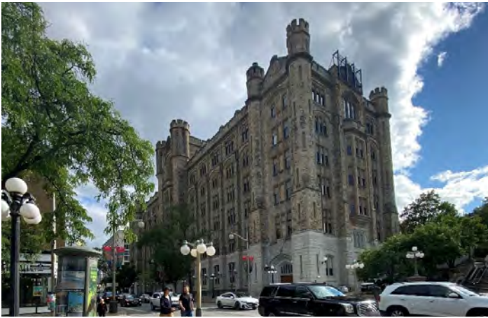
Figure 30: Connaught Building at 555 MacKenzie Avenue
