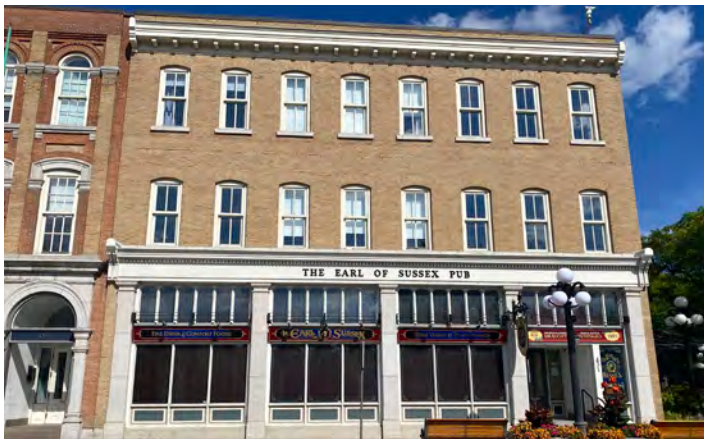
Figure 43: Example of a restored storefront on Sussex Drive.
