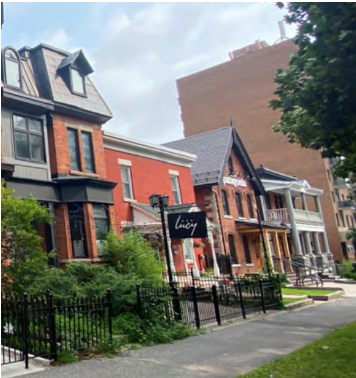
Figure 41: Contributing properties on York Street with a range of porches.
