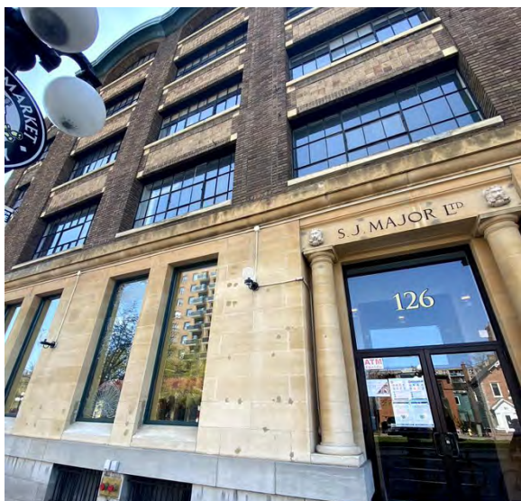
Figure 38: 126 York Street, the Major Building, with its stone and brick materials.
