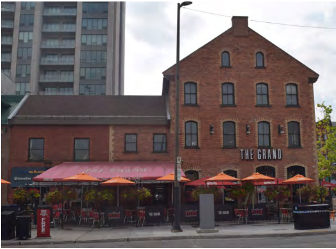
Figure 28: 74-78 George St, former Grand Central Hotel.
