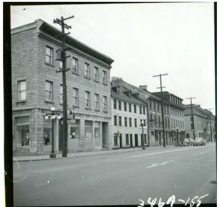
Figure 23: Historic image of Sussex Drive storefronts. Credit: National Capital Commission.
