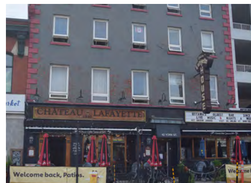
Figure 27: The Chateau Lafayette Tavern at 42 York Street.
