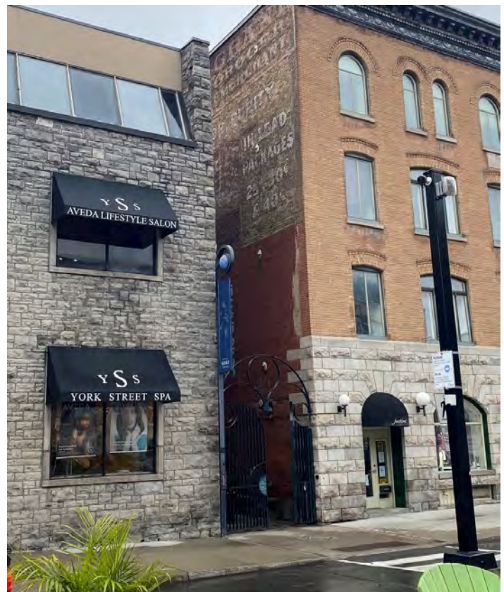
Figure 31: Two buildings on York Street with current awning signs and remnants of a former painted ghost sign.
