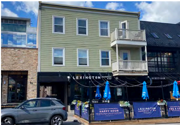
Figure 46: Example of a carriageway that remains at 95 Clarence Street.
