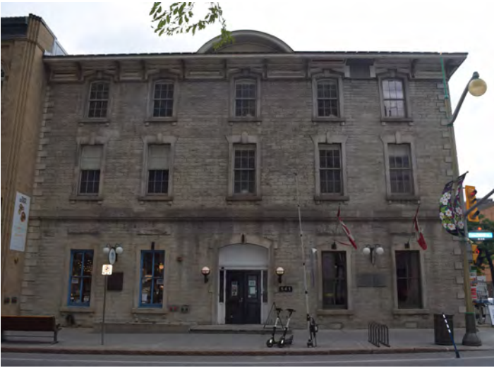
Figure 11: Former Geological Survey of Canada, National Historic Site, at 541 Sussex Drive.
