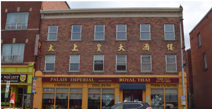
Figure 24: 311-313 Dalhousie Street, brick commercial building.
