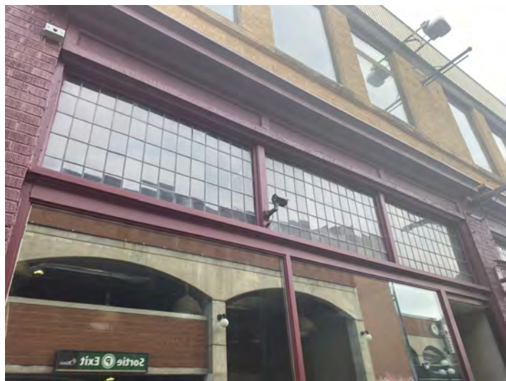
Figure 40: Example of multi-paned leaded windows in the HCD.
