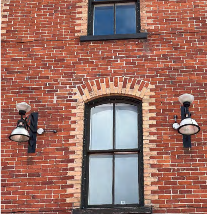
Figure 56: Example of down-facing lighting.
