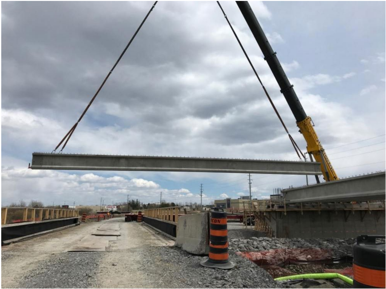
Installation of Bridge Deck Support Frame
