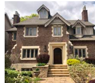
Address: 165 Clemow Construction Date: 1928 Builder: Stewart Christie Company
