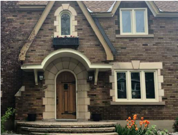
Figure 12: Example of a stone quoining around windows and door
