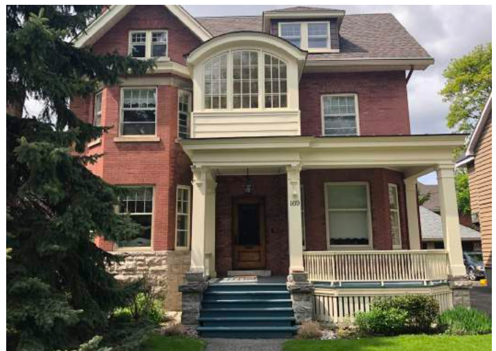
Figure 15: Example of an enclosed upper porch.
