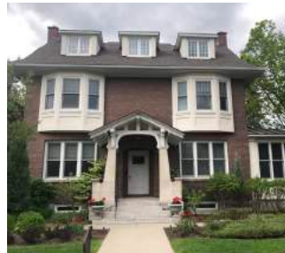
Address: 285 Clemow Construction Date: 1907 Architect: C. P. Meredith
