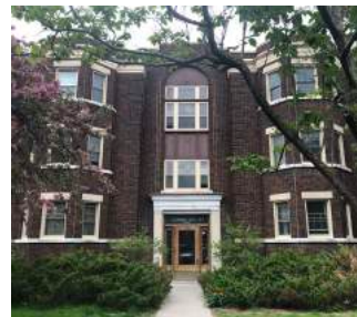
Address: 325 Clemow Construction Date: 1931 Builder: MacDonell & Conyers
