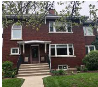
Address: 21 Monkland Construction Date: 1926
