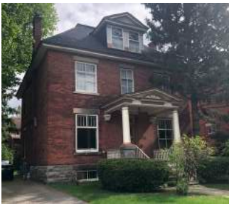
Address: 226 Clemow Construction Date: 1909 Architect: Arthur Le B. Weeks
