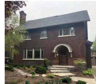
Address: 22 Monkland Construction Date: 1923
