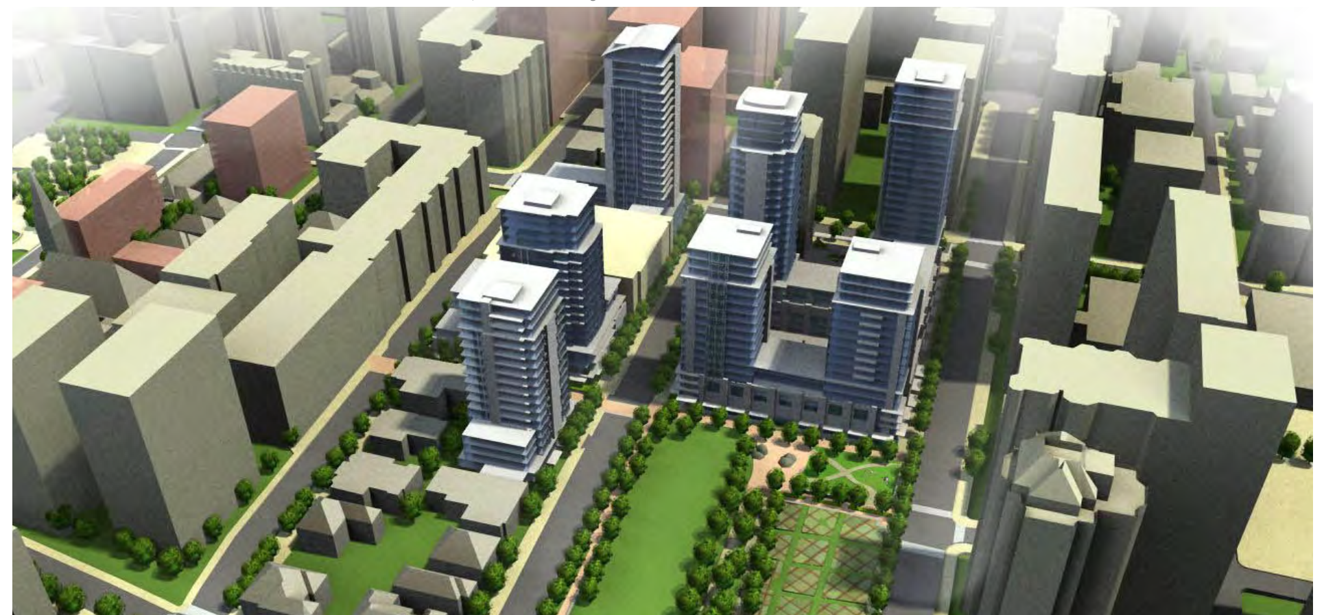
Residential development: OCDSB south site looking west
