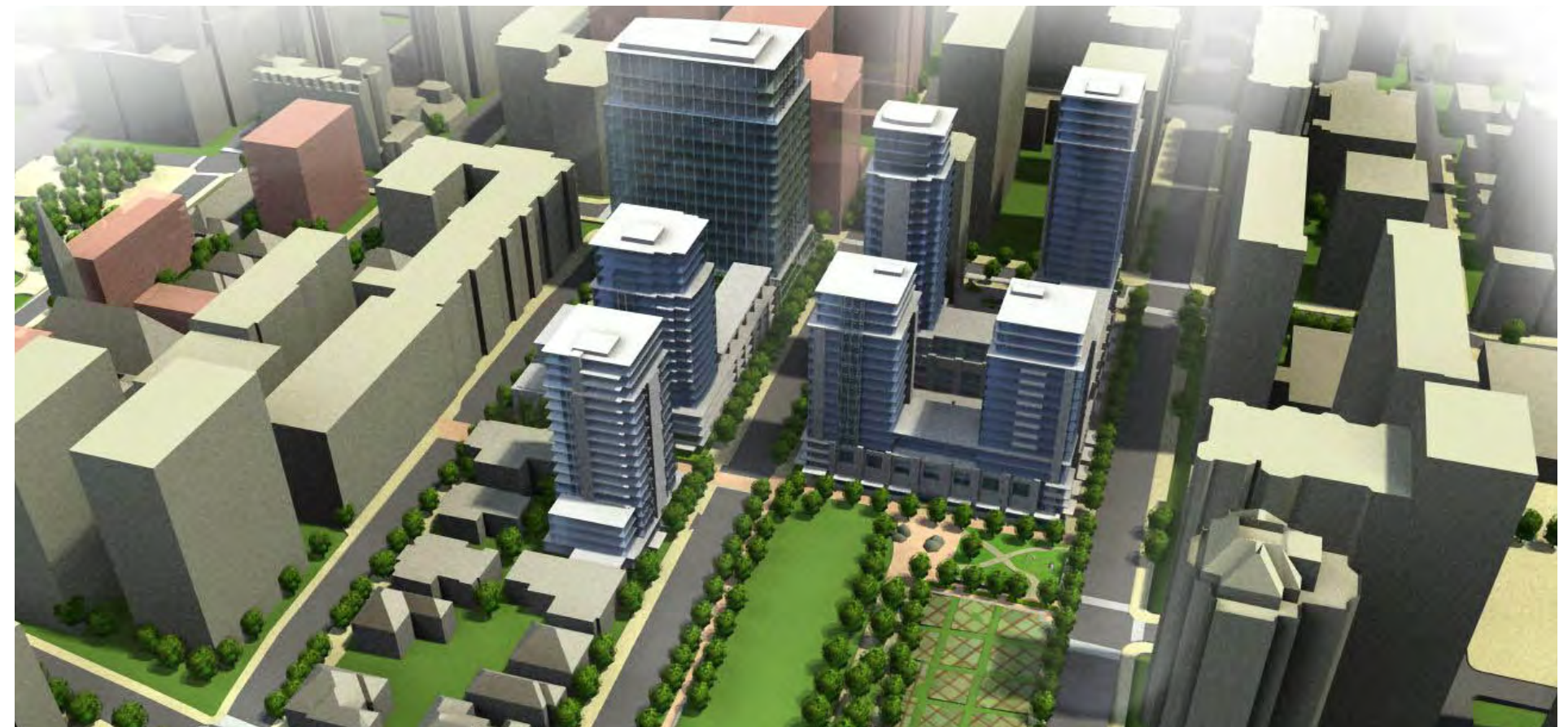
Residential development: OCDSB south site looking west (image to be updated)
