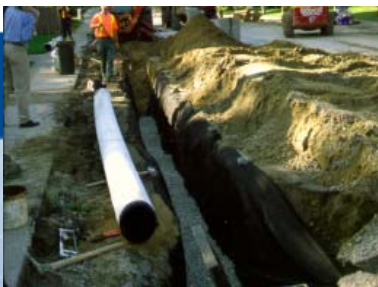
Perforated Pipe (during construction) used to promote infiltration
