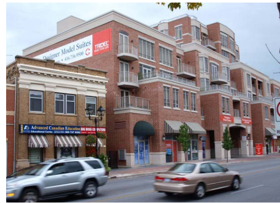
Buildings have wide street frontage and 2-storey street wall is maintained by storey step backs (MMM Group, 2010)
