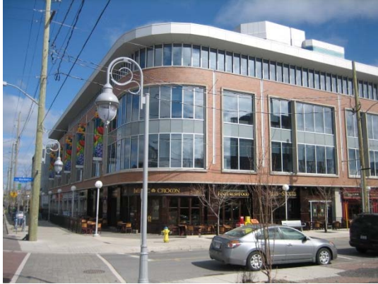
Mixed-use building with street level retail uses (MMM Group, 2011)
