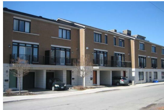
Row housing development in Ottawa (MMM Group, 2011)
