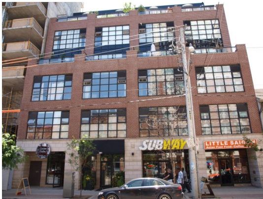
Ground floor animation with step back at the third storey (MMM Group, 2009)
