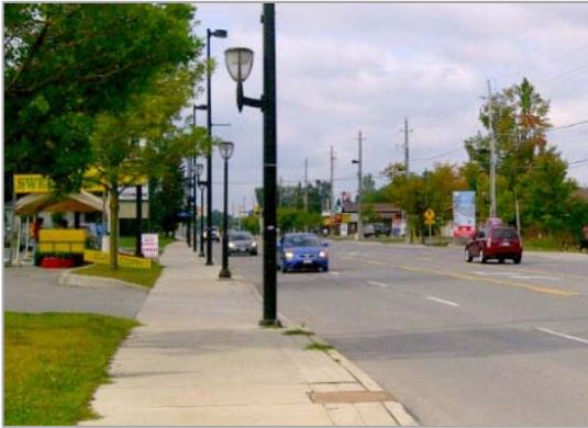
Pedestrian and roadway lighting along Perth Street in Richmond, ON (MMM Group, 2011)
