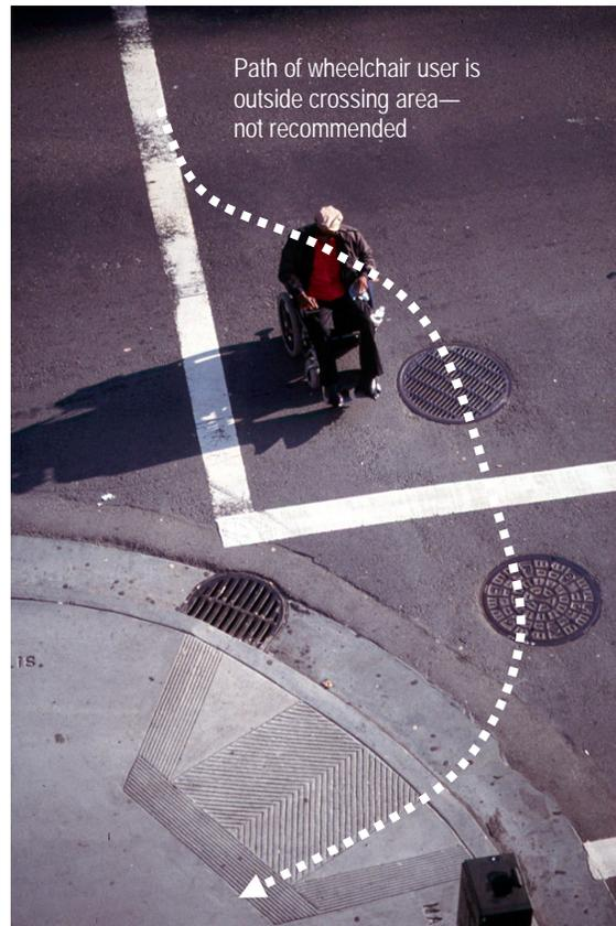
The curb ramp alignment is such that the wheelchair user is directed outside the crossing area in order to access it. Curb ramps must be perpendicular to the curb and should align with the crosswalk Source: [www.pedbikeimages.org](http://www.pedbikeimages.org) / Dan Burden
