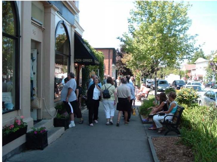
The concrete sidewalk or pedestrian travel zone is uniform in colour and texture with a defined edge, and contrasts with the adjacent zones. Location: Niagara-on-the-Lake, ON. Source: Stantec
