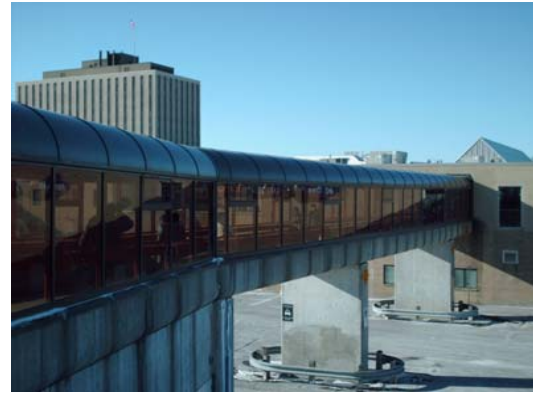
Figure 18: Billings Bridge Plaza is connected to the Transitway by a grade separated pedestrian bridge.
