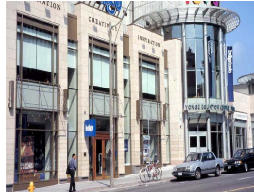
Figure 14: Generous windows with changing displays can both animate the public realm, contributing to quality and interest at transit stops, and benefit the private realm by engaging the attention of transit users passing by or congregating opposite the building.
