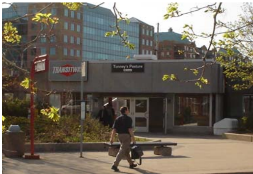
Figure 3a: The Tunney's Pasture Transitway Station is a multi-purpose destination offering a diverse mix of transit-supportive uses that help enable people to meet many of their daily needs, thereby reducing their overall need to travel.
