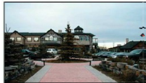
Figure 42: Landscaping along pedestrian walkways buffers pedestrians from vehicles and road spray.
