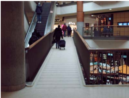
Figure 25: A ramped floor with gradual level changes that meet accessibility requirements is preferred over stairs.
