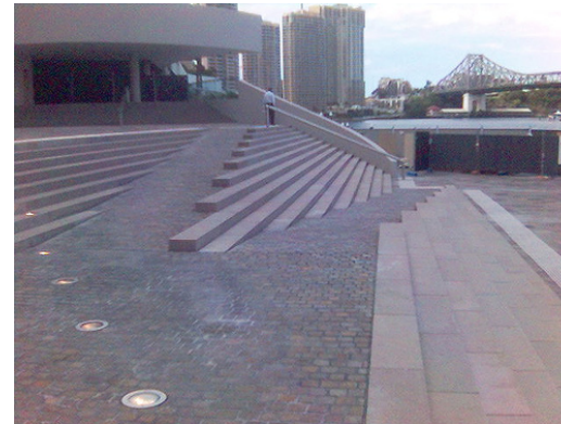
Figure 26: This ramp at the Museum of Civilization is artistically integrated with stairs and provides a levelled area at the top.
