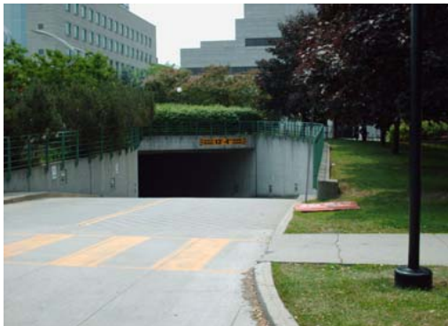
Figure 44: On large sites, loading zones can be located underground to minimize impacts on pedestrians and cyclists. Pedestrians and cyclists should be clearly visible from the loading ramp exit.
