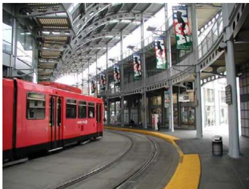
Figure 3b: American Plaza in San Diego is an example of a mixed-use TOD building with uses geared towards both local and non-local residents alike, featuring office space (49 000 m 2 ), retail (2000 m 2 ) and a museum (1000 m 2 ).
