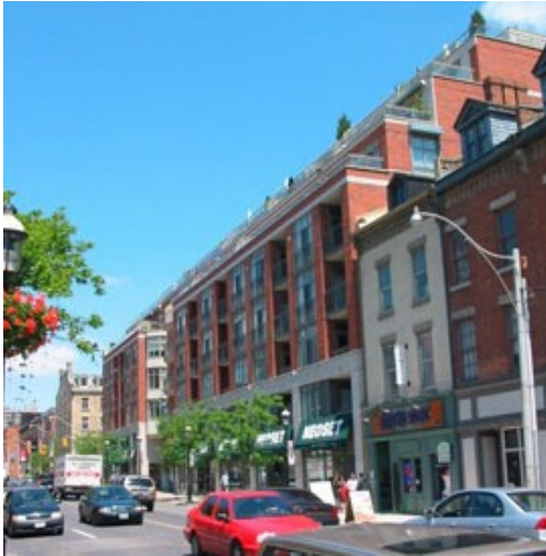
Figure 11a: Buildings set back above 4-5 storeys preserve a human scale and allow more light to reach the sidewalk.
