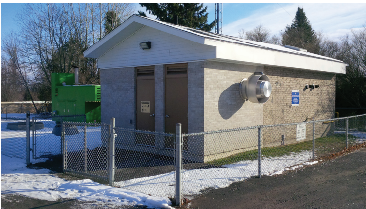
King's Park Pumping Station
