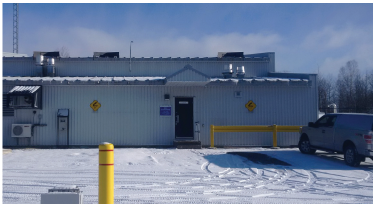
Vars Pumping Station
