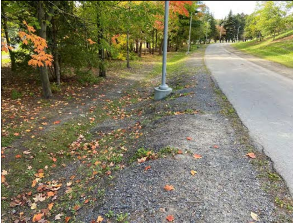
Photo 11: South Drainage Swale: General view of the swale. Road base material has eroded into the swale.
