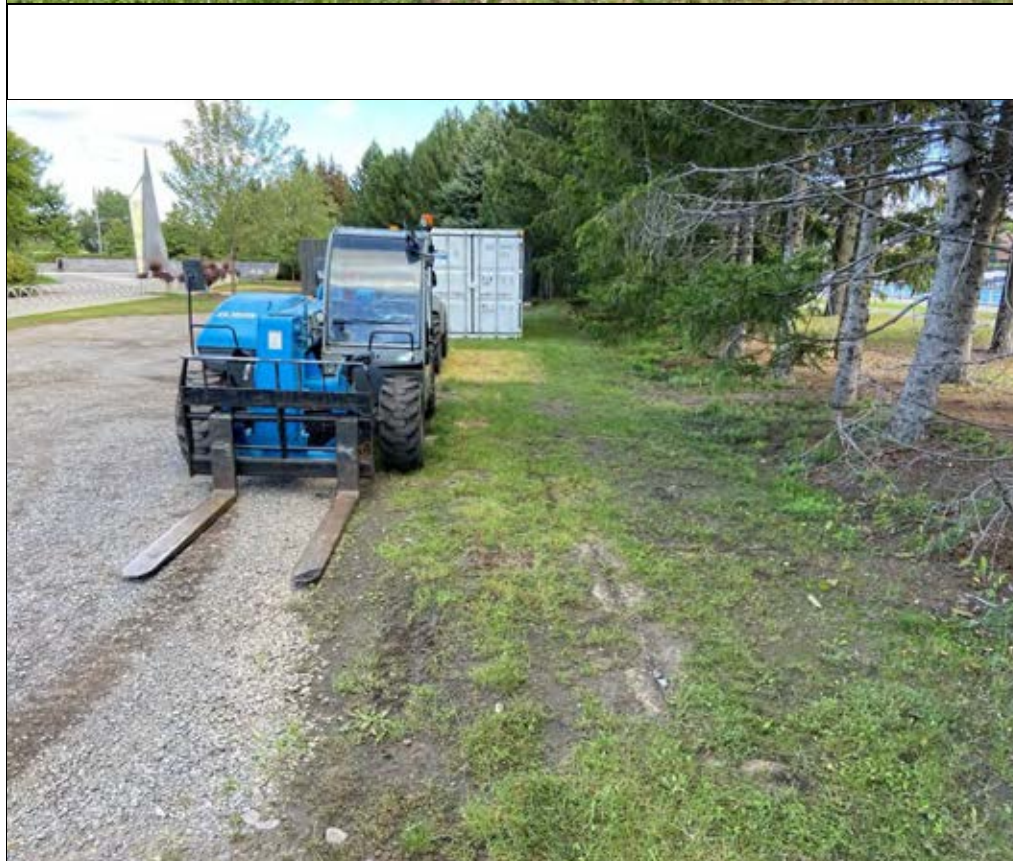
Photo 20: Eastern Perimeter Drainage Swale: Some areas of bare soil and tire ruts were observed adjacent the granular resurfaced area.
