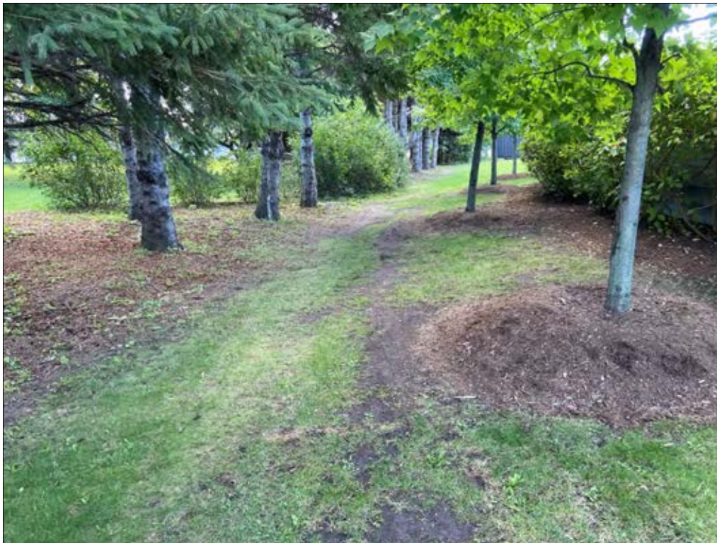
Photo 22: Eastern Perimeter Drainage Swale: General view of the swale east of the Water Plaza. Some areas of bare soil were observed along the property boundary.
