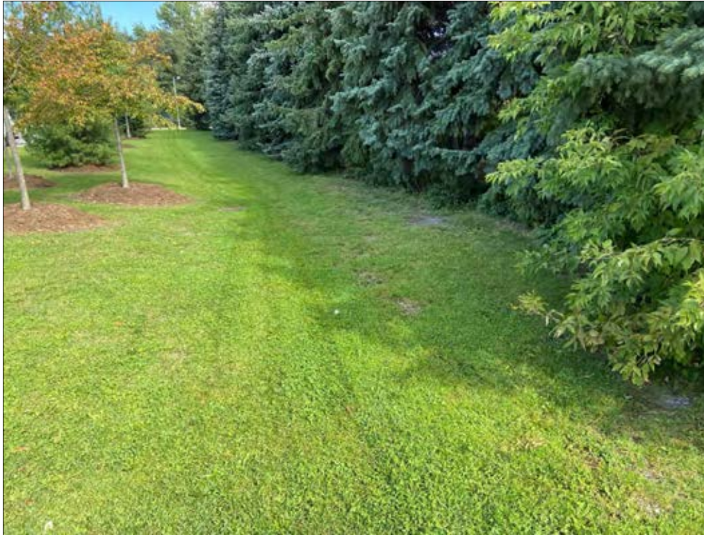
Photo 21: Eastern Perimeter Drainage Swale: General view of the swale east of the Ice Rink and Heirloom Orchard. Small areas of bare soil were observed in the area of the utility trench previously excavated within the swale.
