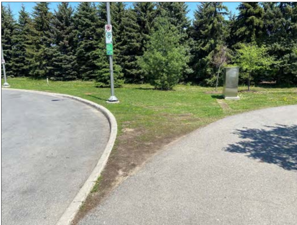
Photo 14: South Drainage Swale: Area of bare soil in high traffic area north of the ice rink.
