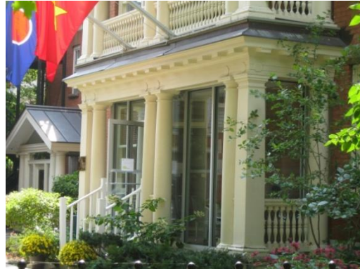
Figure 15: A portion of the porch at 55 MacKay Street was enclosed with glass to provide additional weather protection.
