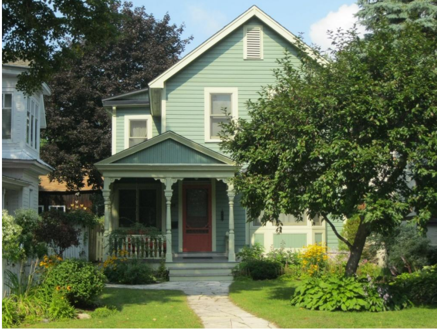
Figure 16: 116 Stanley has a sympathetic addition at the side that does not negatively impact the character of the building.
