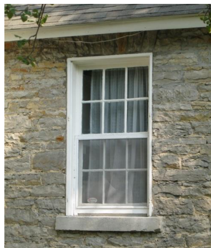
Figure 11: Historic windows were generally sash windows with multiple panes and constructed out of wood.
