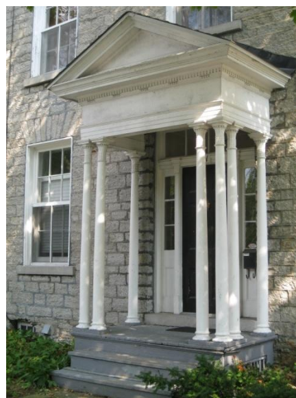
Figure 12: The entrance of this house is characterized by the door, transom window, and sidelights.
