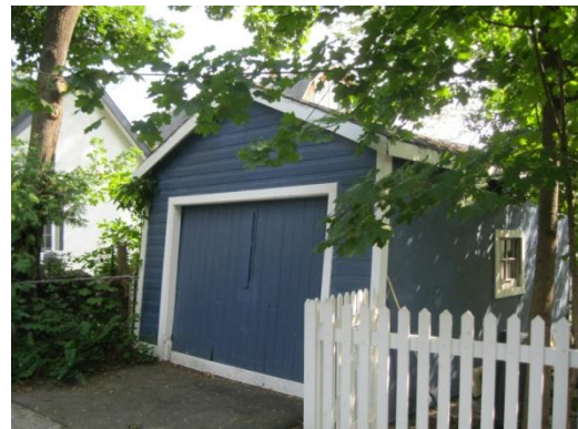
Figure 20: This small garage on River Lane is typical of the small scale wooden garages and former carriage houses found throughout the HCD.
