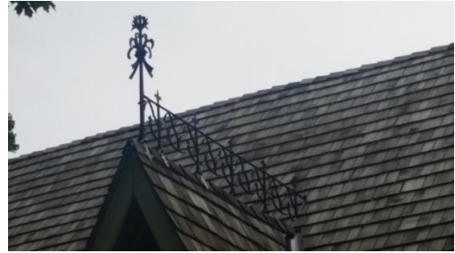
Figure 9: The cedar roof of St. Bartholomew's Church was recently restored.
