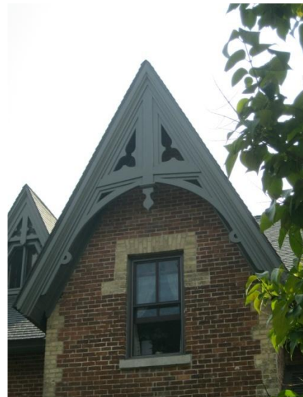
Figure 14: The Frechette House, 87 MacKay Street features decorative bargeboard in the gable ends.
