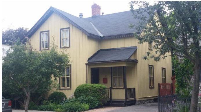
Figure 10: The board and batten wood siding of this house on Crichton Street is an important heritage attribute that should be preserved.
