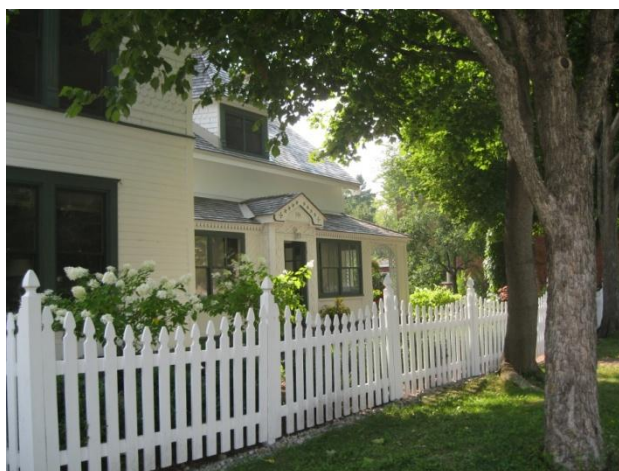
Figure 3: The Bell House is located at 151 Stanley Avenue and is designated under Part IV of the OHA.
