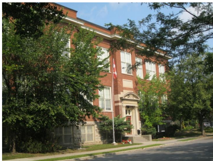
Figure 4: The former Crichton Street School at 200 Crichton Street is an important reminder of the history of New Edinburgh as a self-sufficient village.
