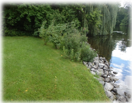
After: Rip-rap installation and buffer planting
