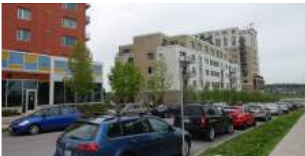
1203 Maritime Way, looking southeast
