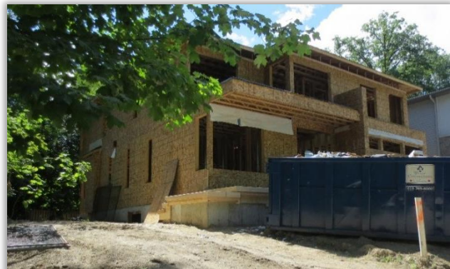
Construction in Queensway Terrace North
