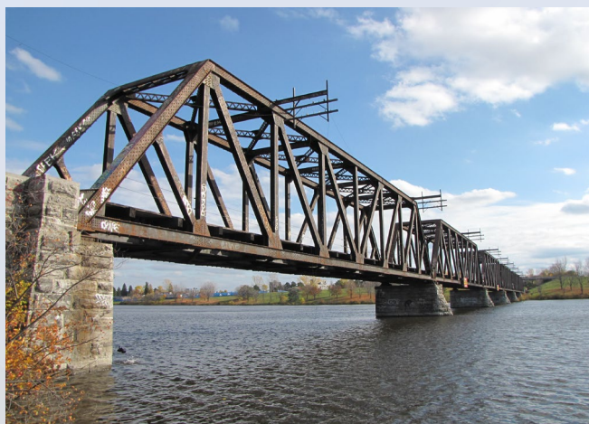
South Bridge, looking south
