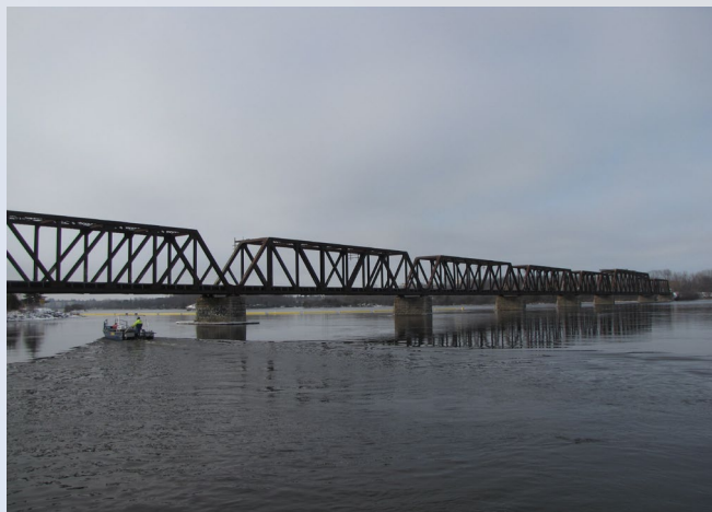
North Bridge, looking north
