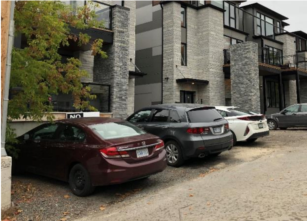
Figure 7: Experience has shown that even if parking is not required, some buildings will end up with cars parked illegally on what should be green space. Physical barriers, required through zoning, can help prevent this.
