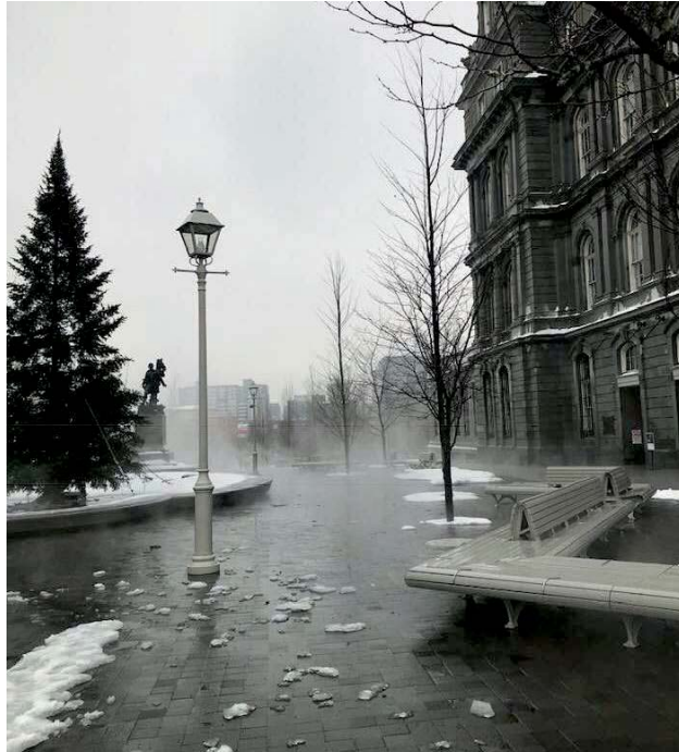
Fig. 138 Heated paved surface near Montreal City Hall Source: Vian
