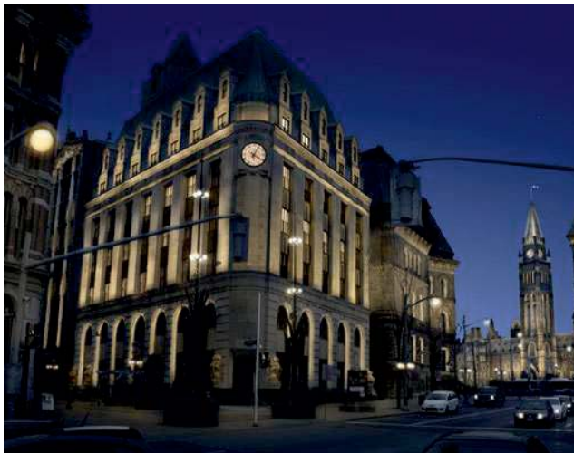
Fig. 62 View of Sparks Street and Egin Street from the east side of Egin Street Source: Parliamentary Precinct Exterior Lighting Master Plan, 2015
