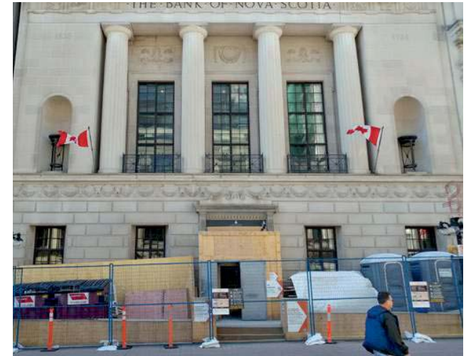
Fig. 25 Construction at the Bank of Nova Scotia Building Source: Vlan + civilti
