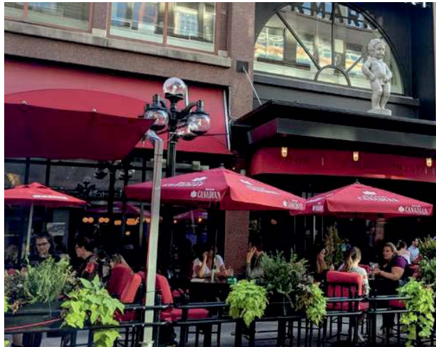
Fig. 47 Biermarket Facade and Patio Source: SSMA
