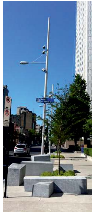
Fig. 94 Multipurpose Streetlight Poles in Montreal Source: Vlan
