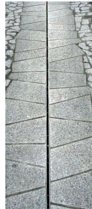
Fig. 142 Stormwater slot drain in paving Source: www.landzine.com/st-four-pavement-by-insitu-landscape-architecture-01.jpg
