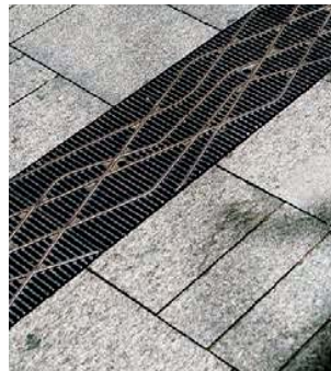
Fig. 140 Technical trench with decorative cover Source: www.landzine.com/index.php/2013/10/pitt-street-mall-by-tony-caro-architecture/
