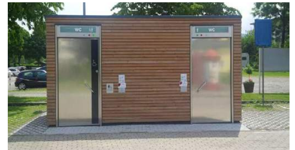
Fig. 119 Toilettes publiques Source: cellcode.us/quotes/ada-design-bathroom-public-compliant.html
