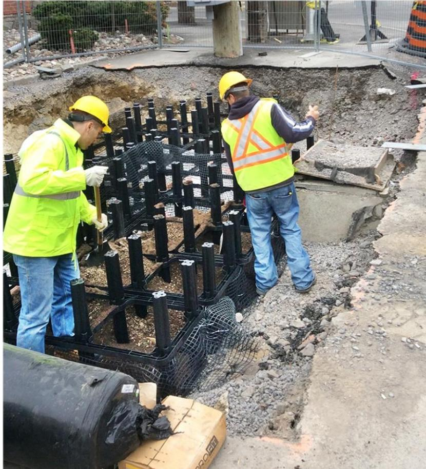
Figure 9: Installation of Silva Cell structural soil cells to provide adequate soil volume for trees along Gladstone Avenue. Image source: Douglas Associates Landscape Architects, 2015 (drcla.ca).
