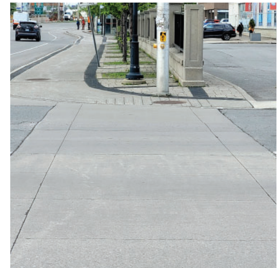
Figure 16: Enhanced pedestrian crosswalk..
