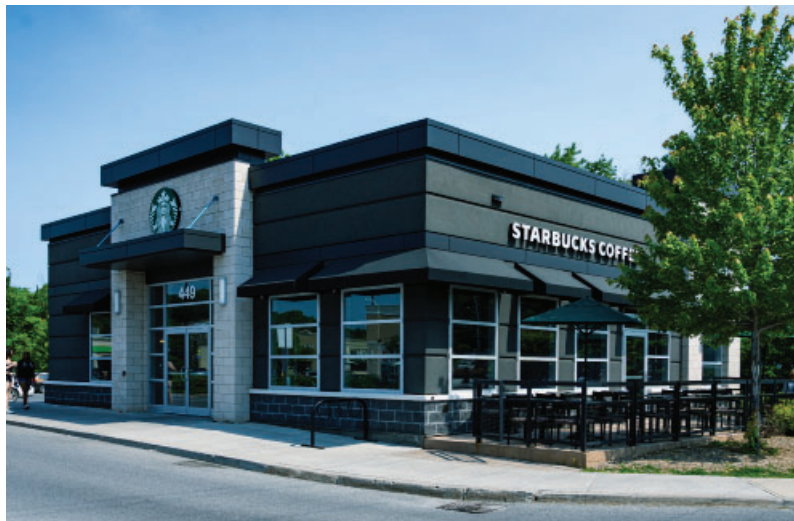
Figure 13: Corporate signs fit with the design and scale of the building.
