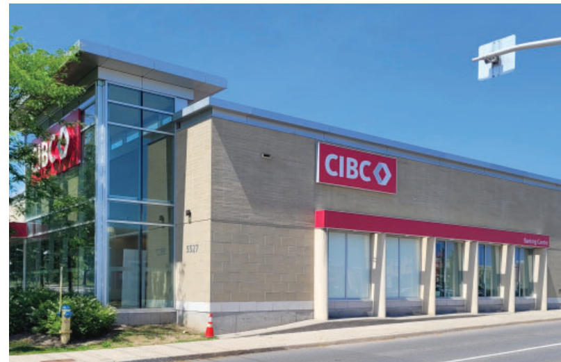
Figure 14: Wall projections and colour/material changes reduce the perception of building size.
