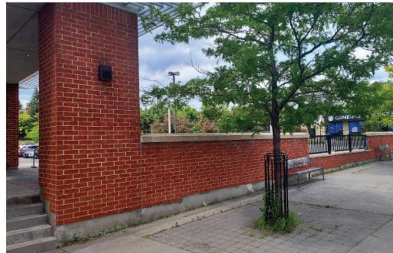
Figure 22: Low wall screens the parking area, mitigates the grade difference, and defines the edge conditions of the development.
