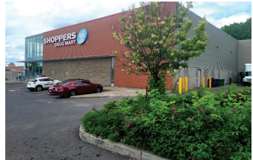
Figure 8: This development locates loading docks, ramps, garbage and recycling containers at the back of the site.
