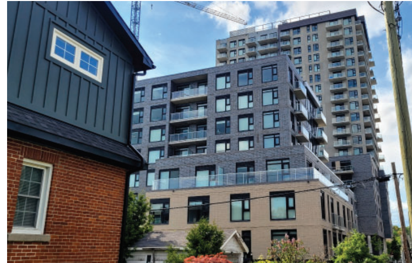
Figure 10: The transition strategy of this development includes progressive reduction of heights, and massing and facade articulations.
