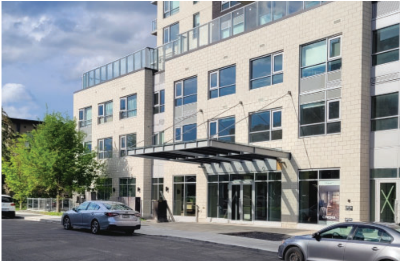
Figure 9: The podium of this development supports the creation of continuous streetwall with appropriate street section ratio.
