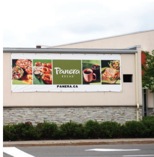
Figure 2: At the back of this drive-through restaurant, architectural details are consistent with the other sides of the building.
