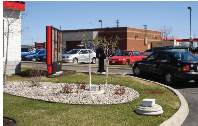
Figure 27: The planting area collects and stores stormwater.
