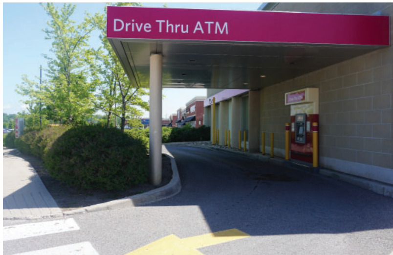
Figure 15: The ATM of this drive-through bank is directly visible from the surrounding areas, providing a sense of security for users. .
