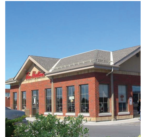
Figure 3: This drive-through development responds to its traditional village context using a compatible building style.
