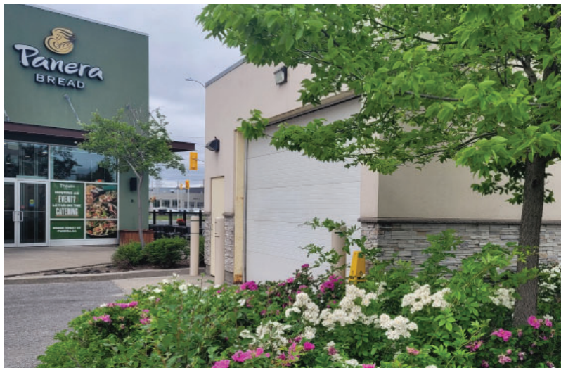
Figure 21: The overhead pergola and landscape along the edge of the site screens the driveway from street.
