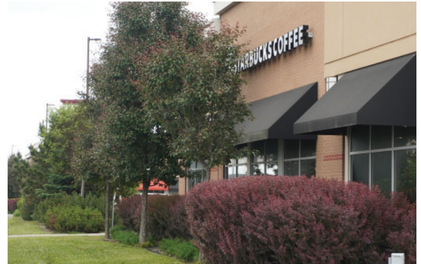
Figure 18: Awnings, foundation plants, trees and different color of the drive through facing the public street adds animation.
