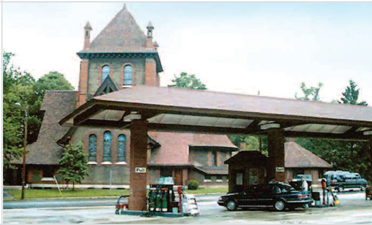
Figure 1: The architectural treatment of this gas station canopy reflects the context.
