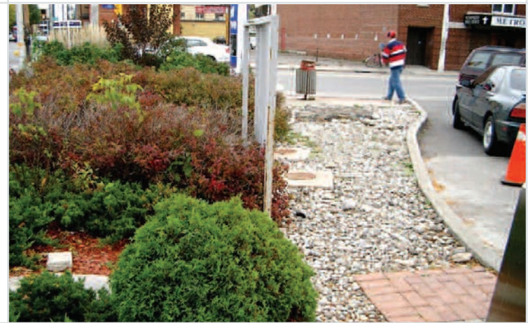
Figure 18: The planting island collects and stores stormwater.
