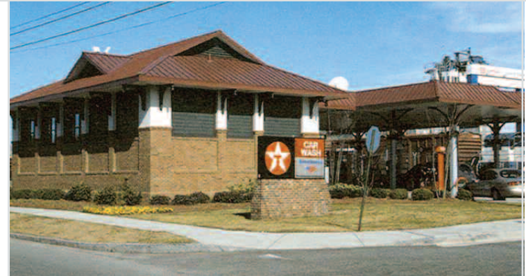
Figure 2: A convenience store close to the street contributes to a well-defined street edge.
