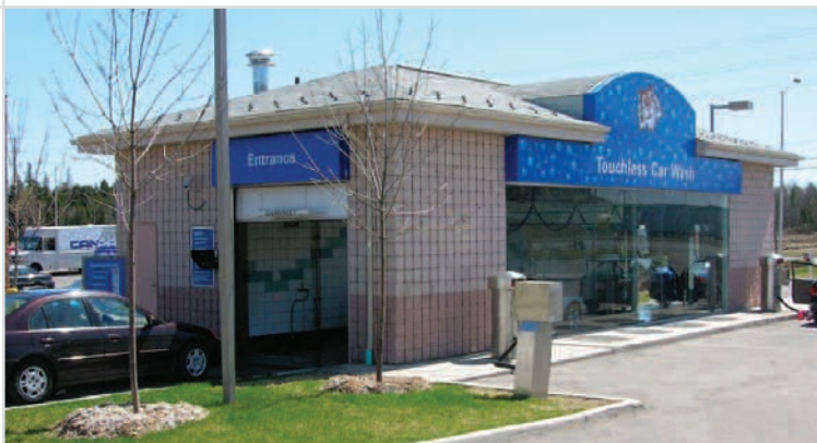
Figure 5: The glass windows of this car wash face the public areas.
