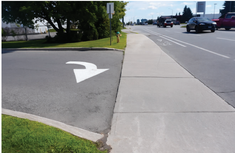
Figure 10: The width of driveway is wide to avoid conflict with pedestrian along the street.
