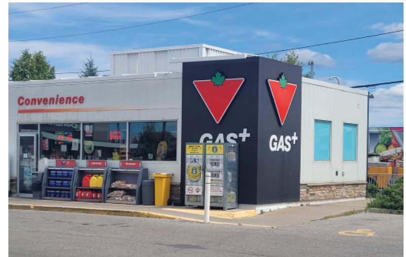
Figure 2: A convenience store close to the street contributes to a well-defined street edge and provides direct pedestrian connection.
