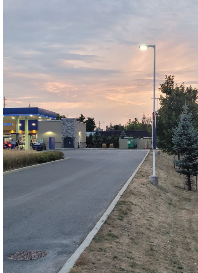
Figure 21: Lighting does not affect the surrounding and provide enough light to the service.
