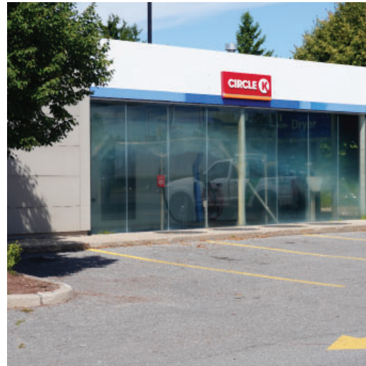
Figure 4: The glass windows of this car wash face the public area.
