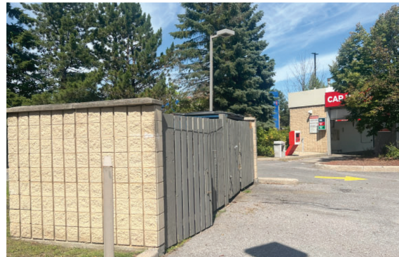
Figure 13: At this gas-station, the garbage enclosure structure is visually harmonized with the main building through similar material colour and texture.
